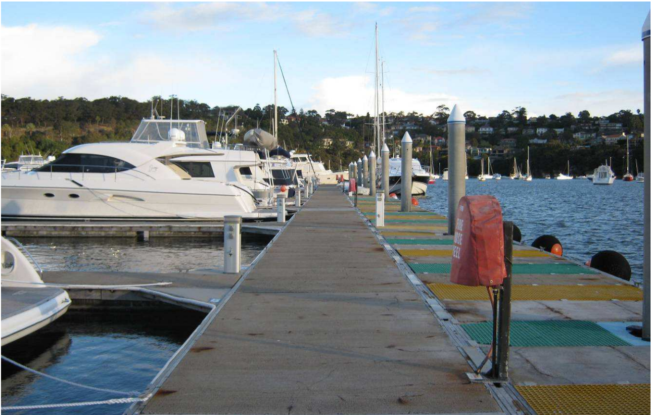
Figure 15: Existing Arm C illustrating pontoon and piles (Source: photograph by department)
