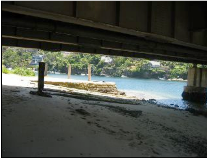
Figure 2: Southern stone punt ramp, exposed at low tide. Source: WP Architects.
