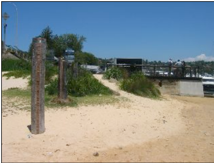
Figure 6: The line of timber piles below the end of the vehicular turning circle denotes the eastern side of the first bridge.
