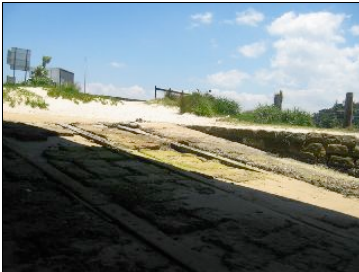
Figure 3: The southern stone punt ramp below the west-bound road lanes of the present Spit Bridge. The sandstone blocks are set between parallel timber beams. Source: WP Architects.
