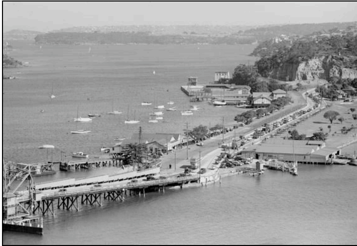
Figure 9: View to the first Spit Bridge, taken in the 1940s.
