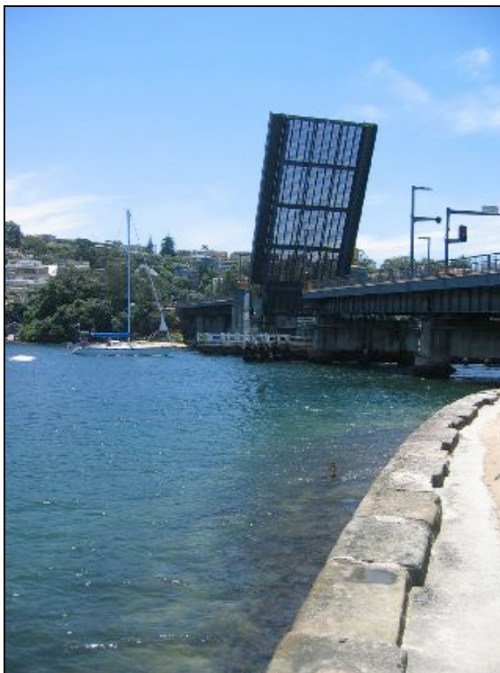
Figure 14: The Spit Bridge, with bascule span raised to allow a yacht to motor downstream.
