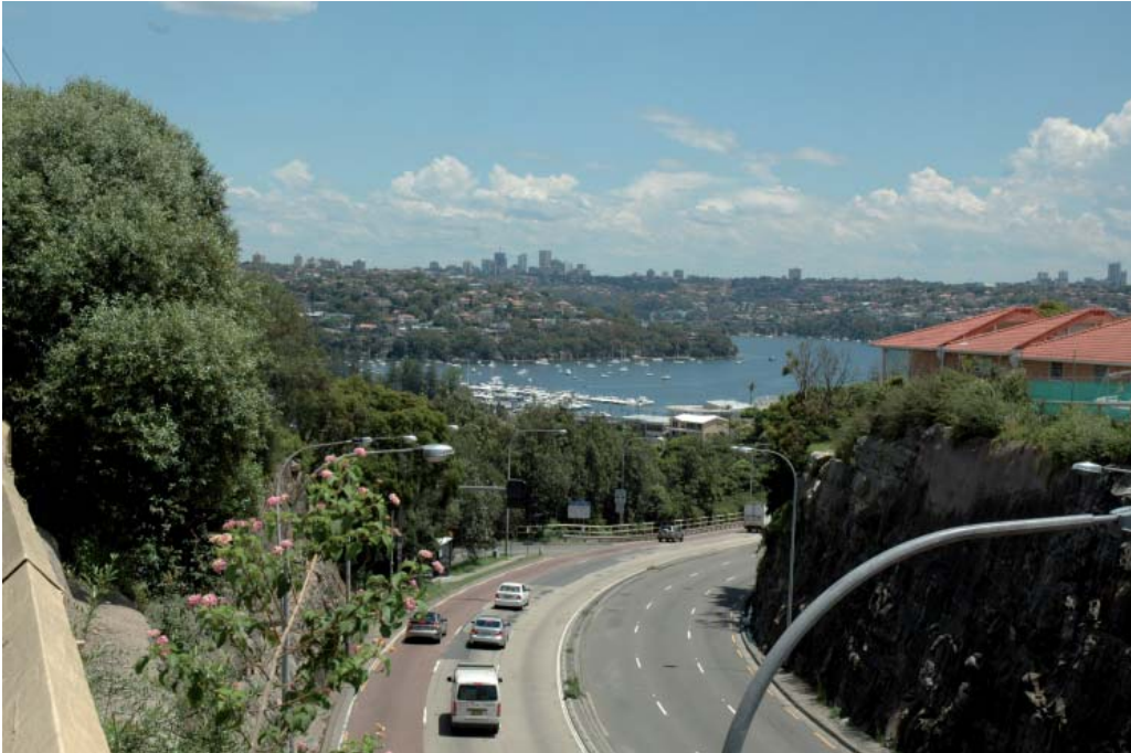
VP3, from north of 19 Kanangra Crescent (near intersection of Kanangra Crescent and Ethel Street), Balgowlah Heights, looking southwest
