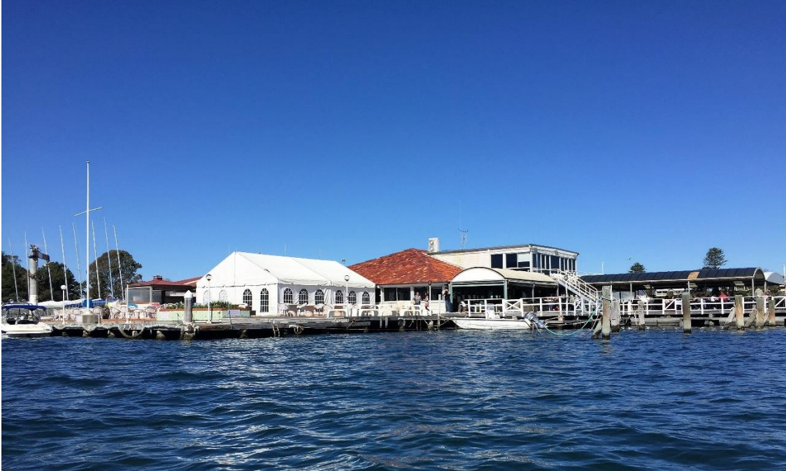
Image 7 BEFORE – View from Lake Macquarie. Existing Marquee in place.
