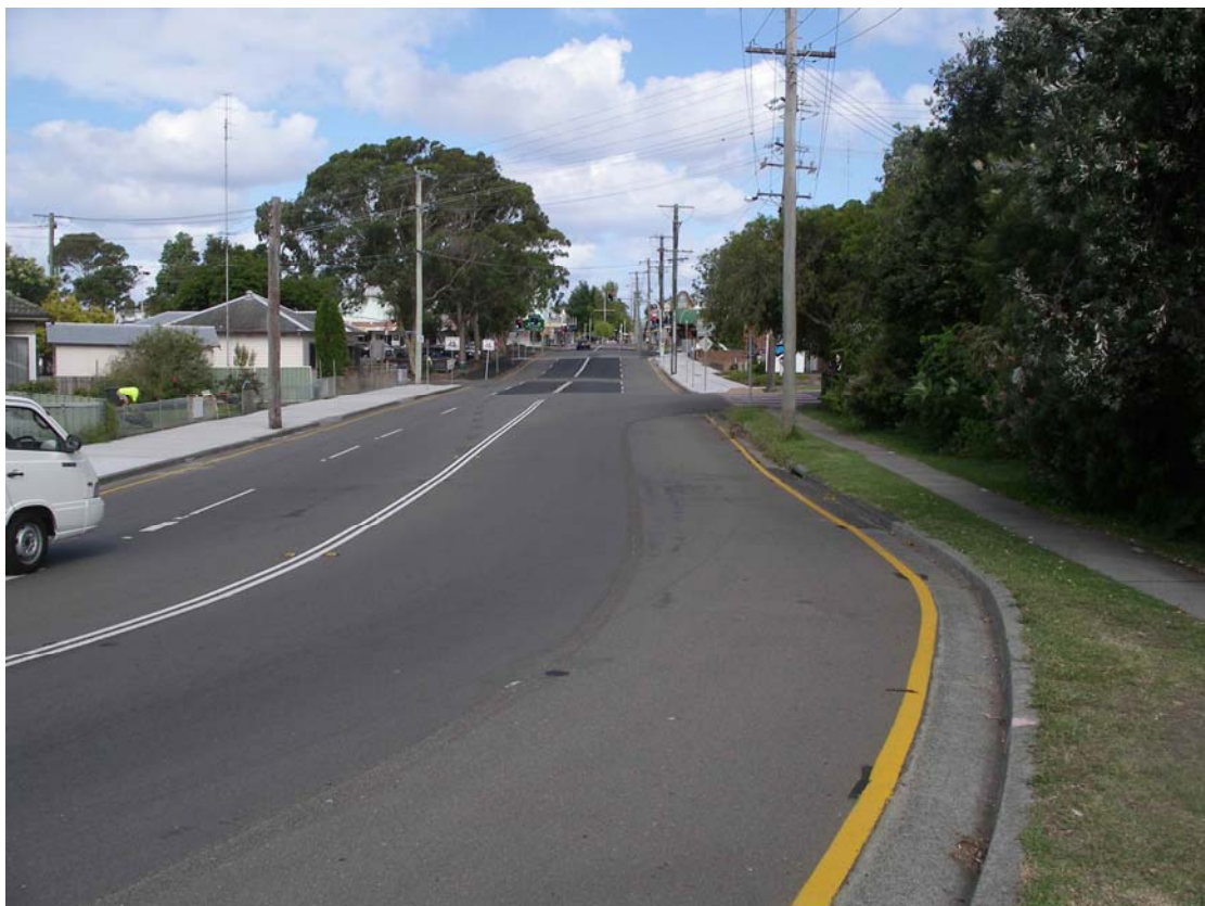
Photo No. 4: Looking generally east along Macquarie Street from Brooks Parade showing the existing traffic environment and the junction with Walter Street on the right.
