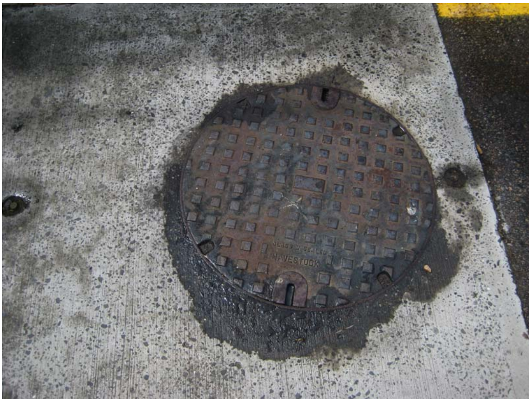
PHOTO TEN: Surface evidence of kitchen oil sump (AEC 4)
