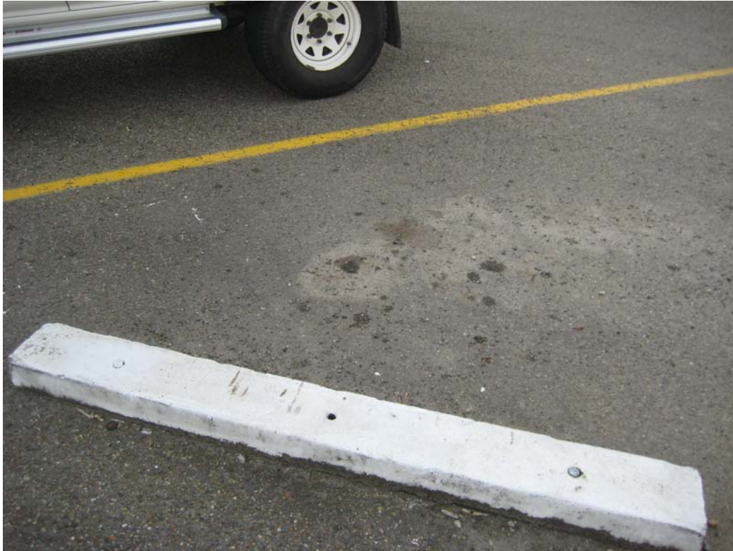
PHOTO FIVE: Example of oil staining in the bitumen car park (AEC 2).
