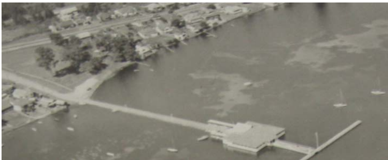
Plate 2 Circa 1950's view of boatsheds and jetties, note their proximity to the water line. Also note the low sandy beach now filled and extended for the car park.
