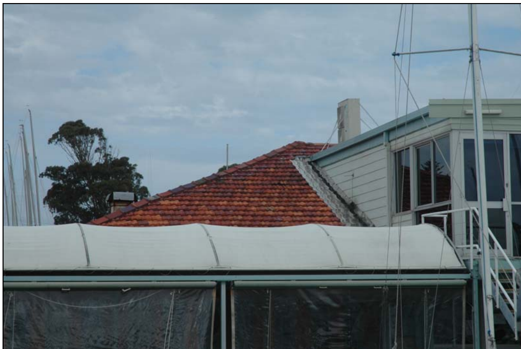
Photo 6 South east corner roof modifications.
