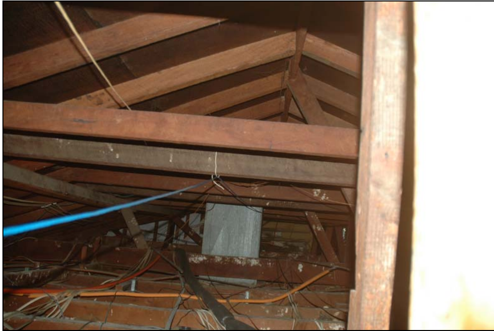
Photo 11 Replacement trusses in the ceiling
