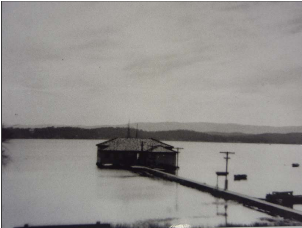
Plate 5 LMYC no date, but prior to jetty widening and installation of awning at entry, prior to 1959 (Ref 0488).
