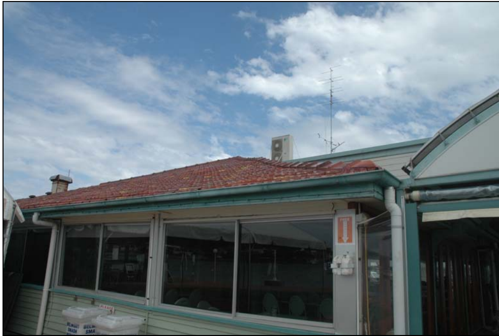
Photo 9 Aluminium window that do not match the original period of construction
