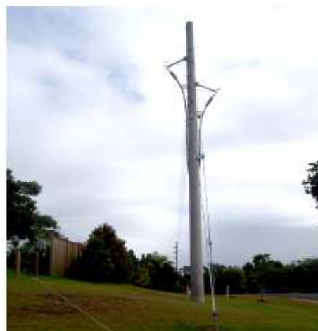
Figure 23 - Example of Overhead to Underground Transition Infrastructure
