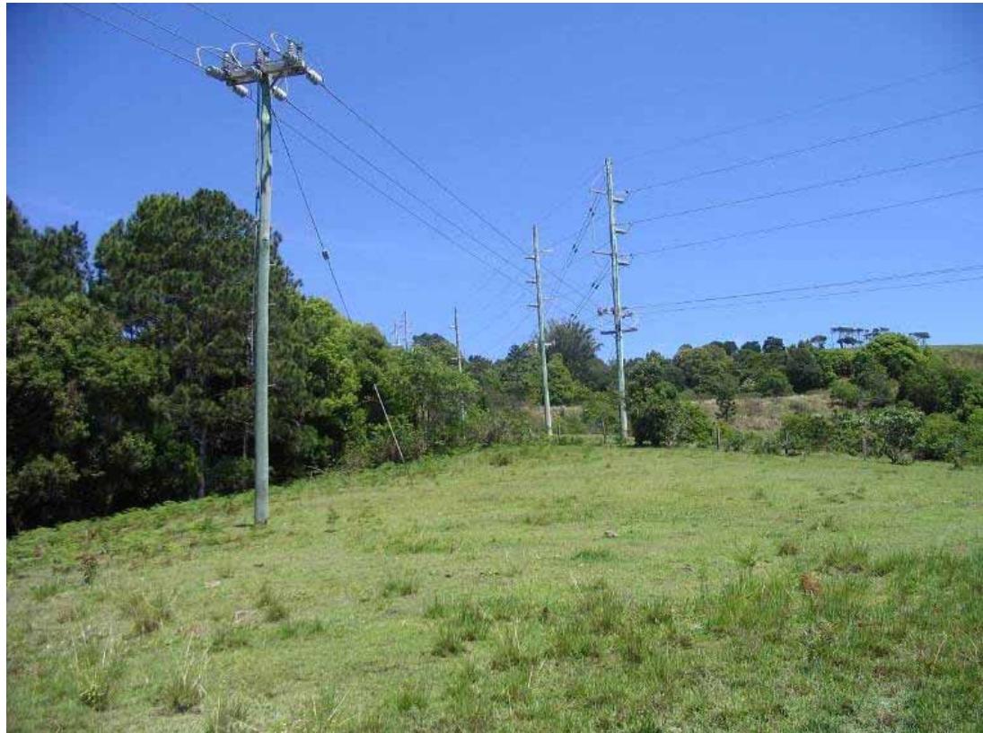
Figure 3-5: View looking south-west from Site 7 along existing 66 kV line.
