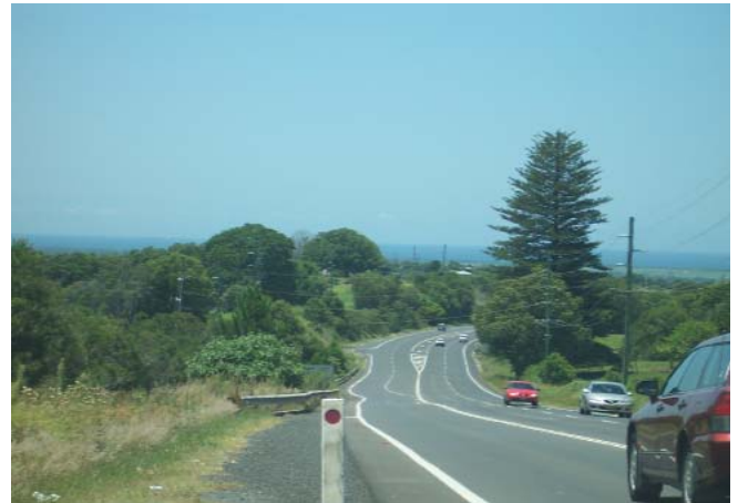
Existing 66kV powerline along the Bruxner Highway
