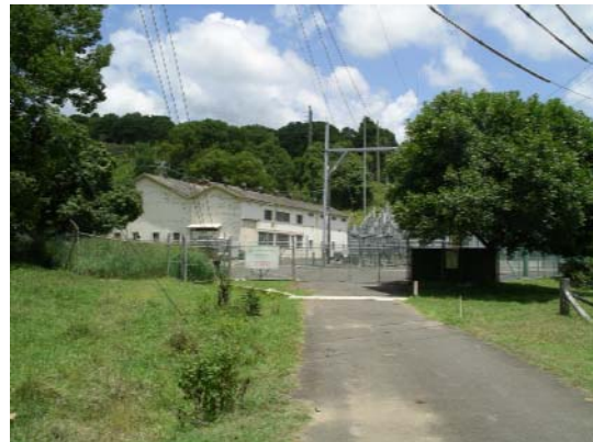
Mullumbimby Zone Substation and old power station
