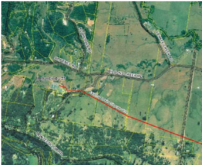
Aerial view of Lavertys Gap and Mullumbimby Zone Substation
