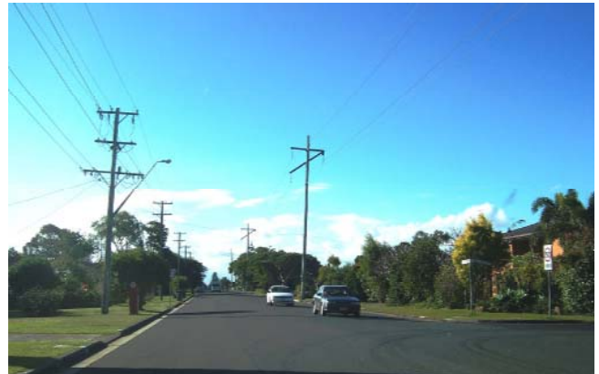
Existing 66kV infrastructure in Alstonville
