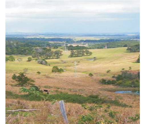
Existing 66kV corridor near Byron Bay
