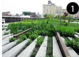
1 paving feathered into turf area
