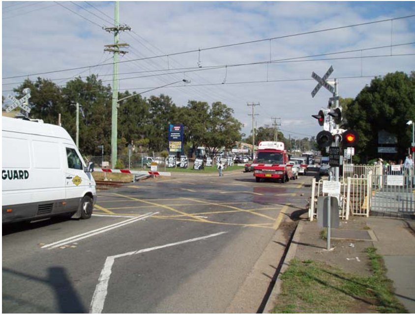
Photograph 5-3 Garfield Road level crossing at Riverstone, facing west
