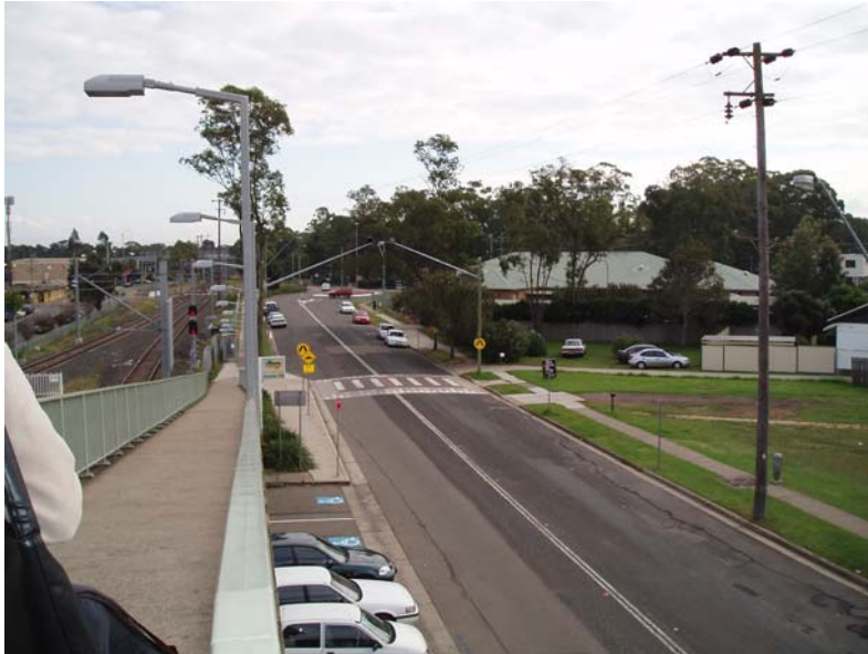
Photograph 5-5 Quakers Hill Station, facing north
