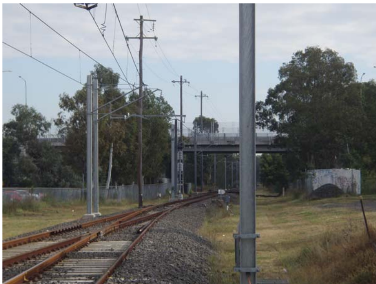
Photograph 1-1 The end of the duplicated track, just north of Quakers Hill Station, facing Quakers Hill Parkway (overbridge)
