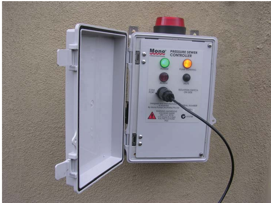
PSS Eco 1-60 Controller (shown connected to Hand Held Display / Diagnostics Unit)
