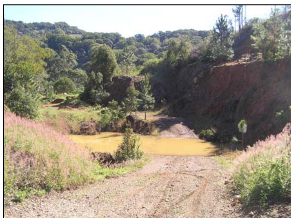
Plate 3. Dam located on western portion of site
