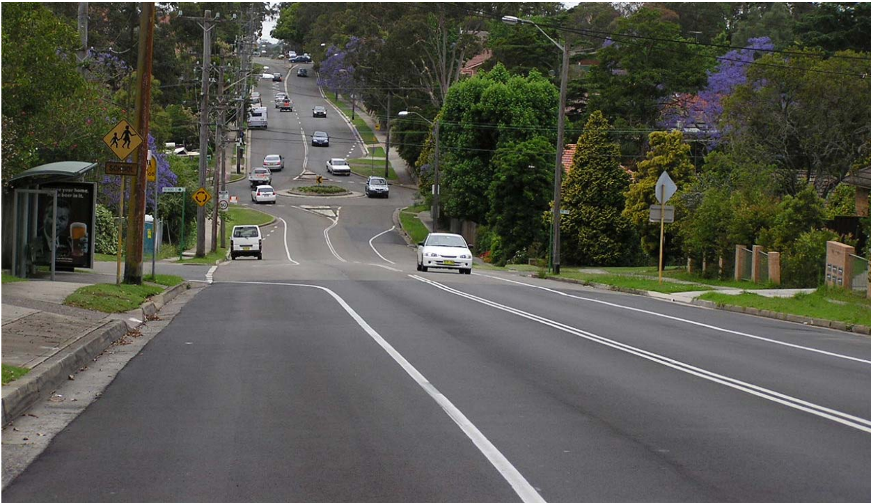
Photograph 3.5 Balaclava Road looking south
