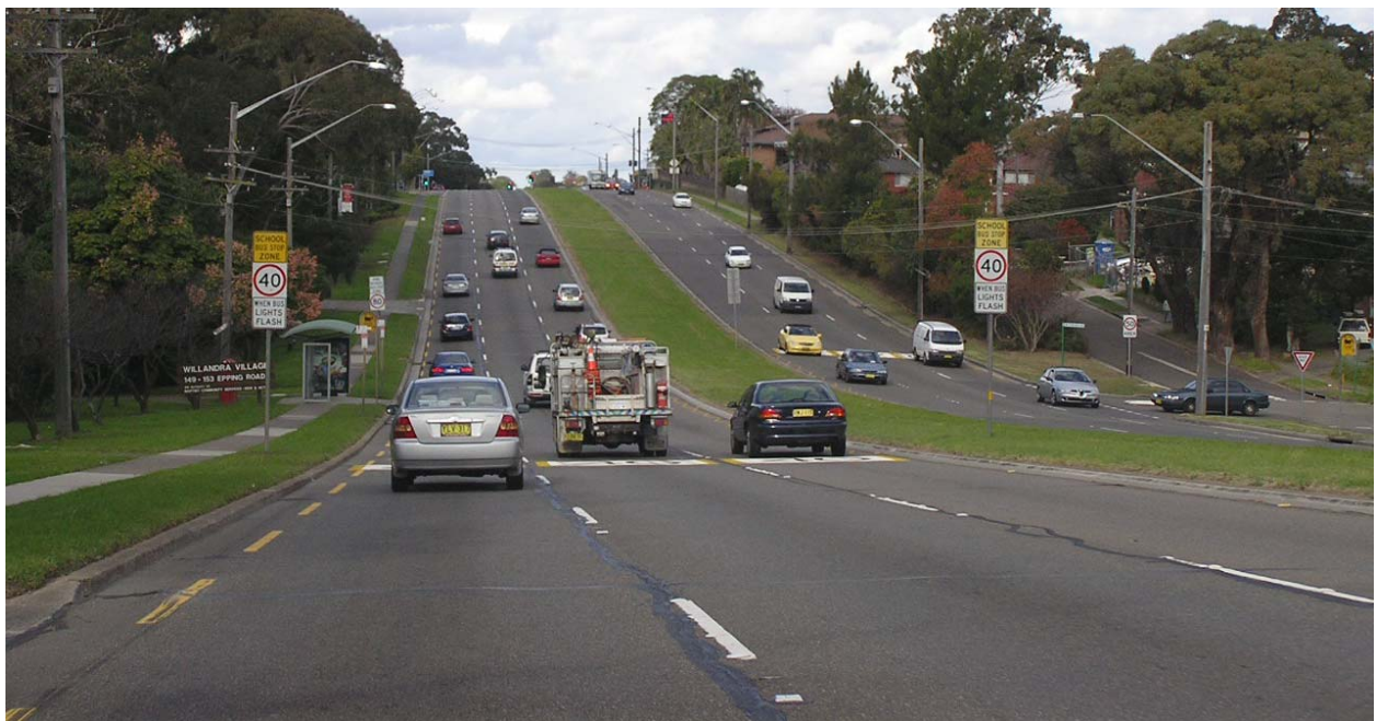
Photograph 3.1 Epping Road looking east
