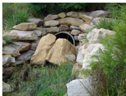
PROPOSED NATURAL ROCK RIP RAP AT INLET
