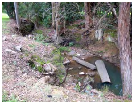
EXISTING INLET STRUCTURES
