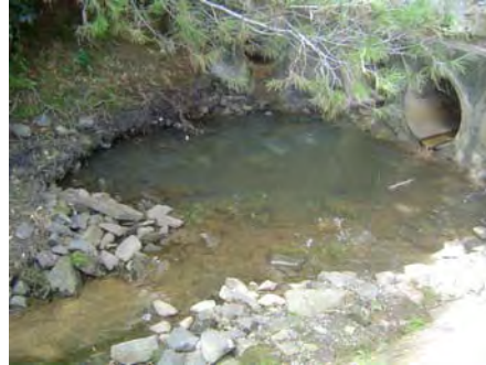
EXISTING INLET STRUCTURES
