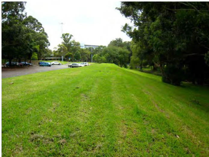
VIEW LOOKING NORTH FROM WITHIN SITE TOWARDS FUTURE RIPARIAN AREA AND CAR PARK
