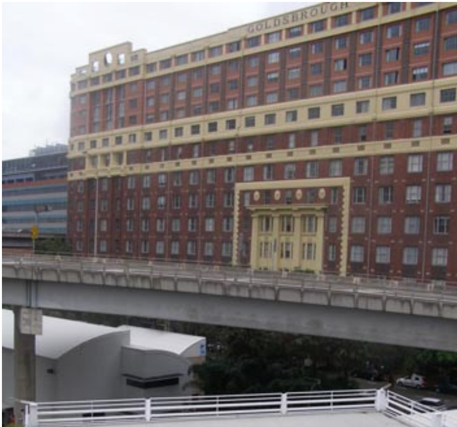
Figure 4 – Western Distributor and Goldsbrough apartments
