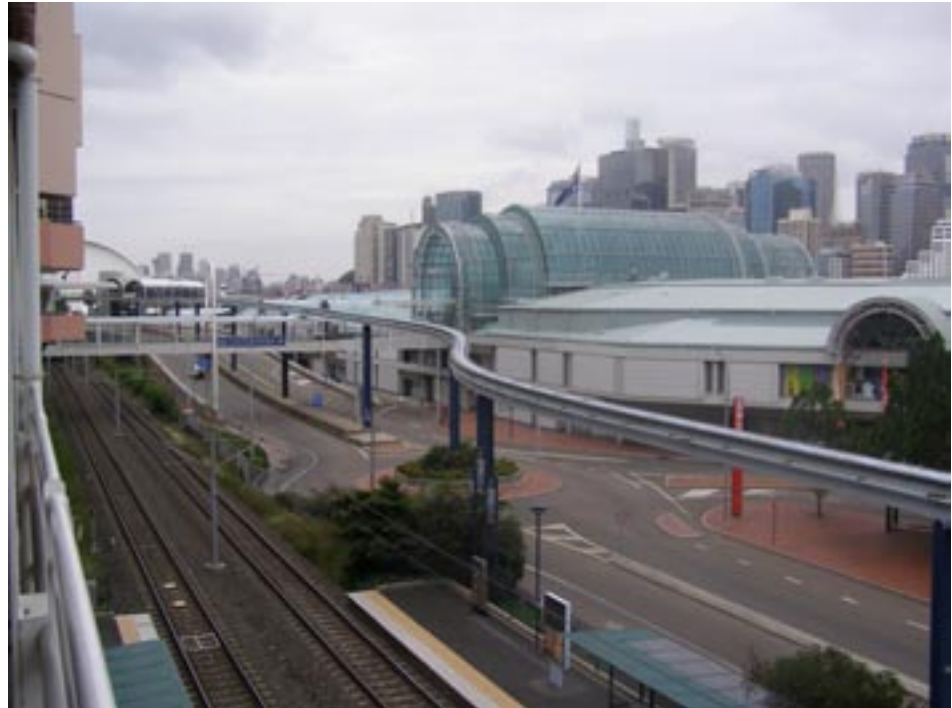
Figure 5 – Lightrail, monorail, Darling Drive and Harbourside Shopping Centre to the east of the site
