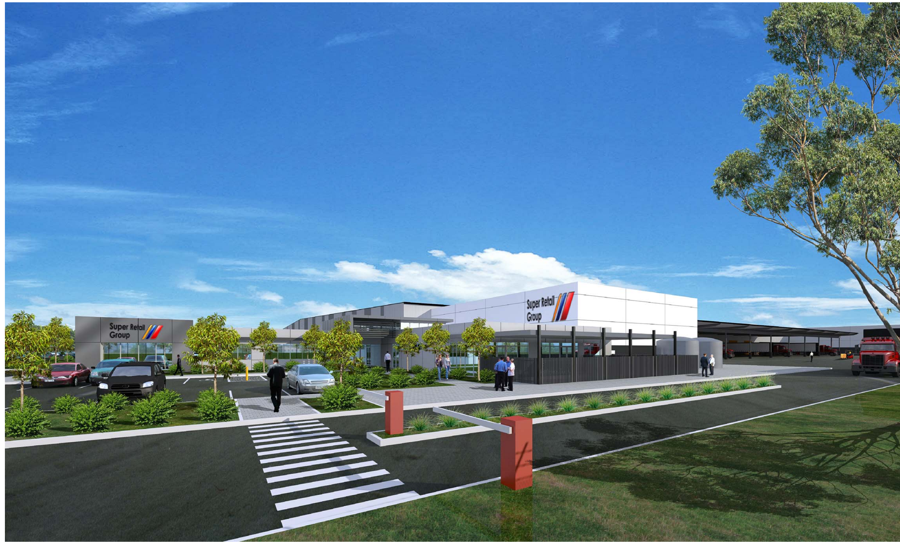
VIEW FROM SOUTH EAST CORNER OF SITE
