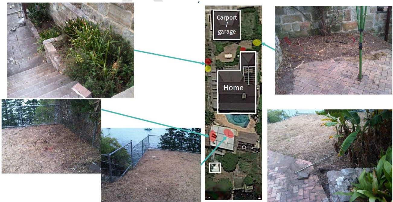
Figure 3: Private Property Works 5 Nelson Parade (excavation areas shown in red and yellow dots)
