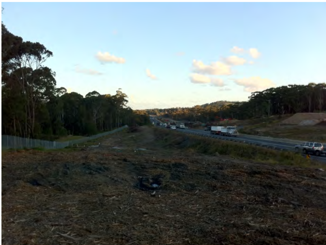
Photo 4 The land to the west of the site, including parts of the subject land acquired by the RTA, which has been cleared as part of the Pacific Highway upgrade.
