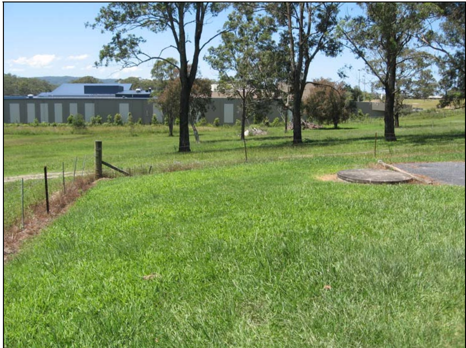
Photo 12: Septic tank and disposal fields.
