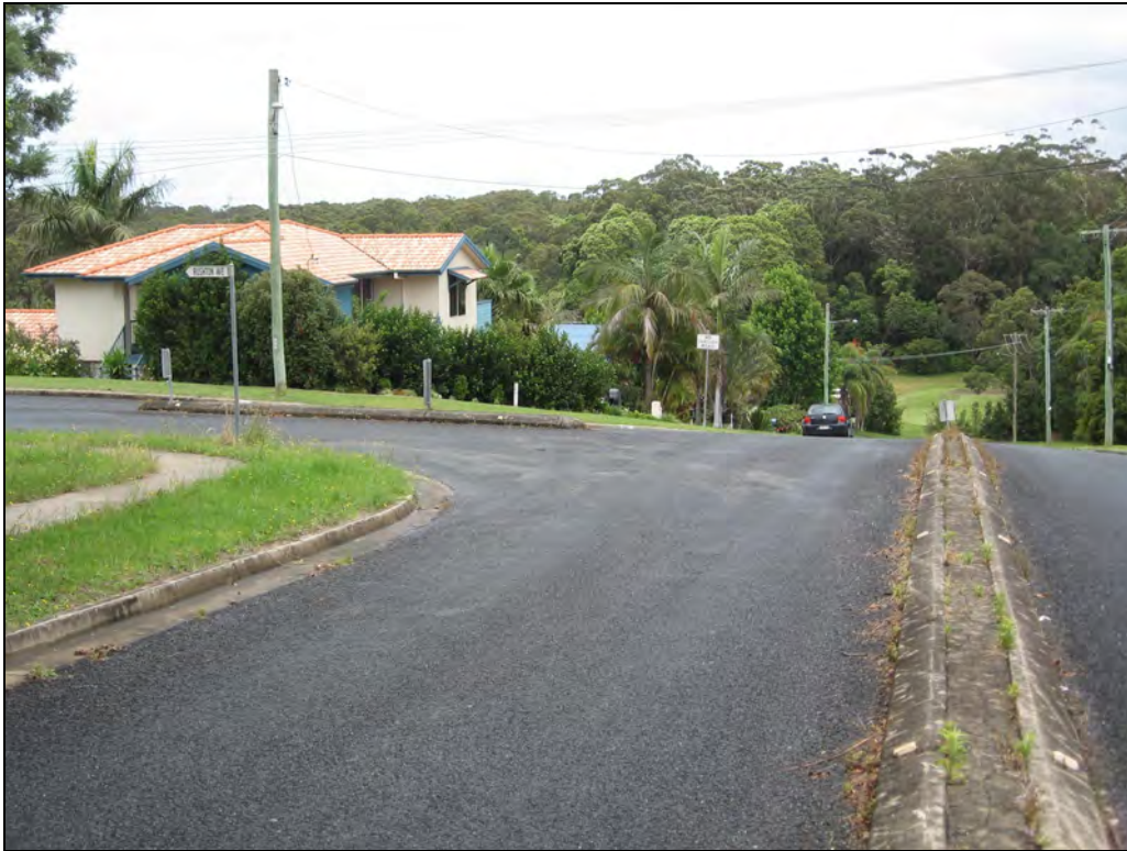
View of narrow section of Woodhouse Road looking south
