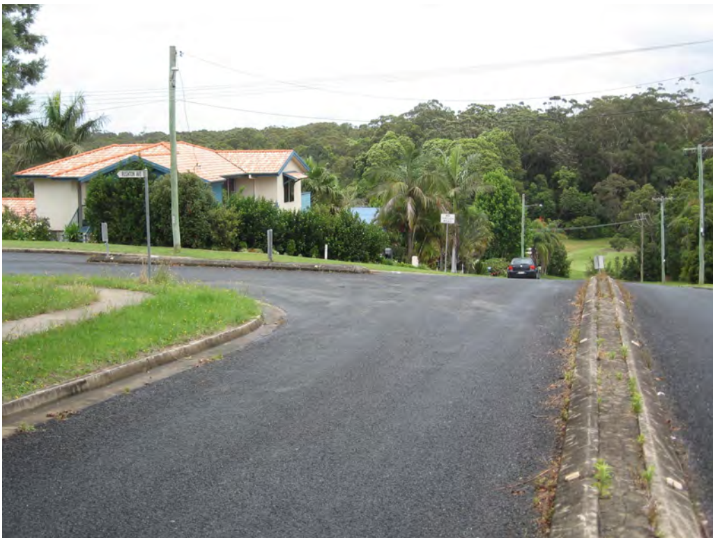
Photograph 1: View of narrow section of Woodhouse Road looking south
