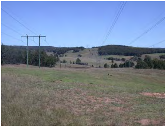
Photo Location 5 – View west from Canyonleigh Road along existing transmission line corridor. Views toward the proposed Facility are blocked by a combination of landform and vegetation.
