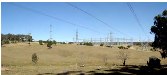
Photo Location 8 – View south from existing transmission line easement toward TransGrid switchyard.
