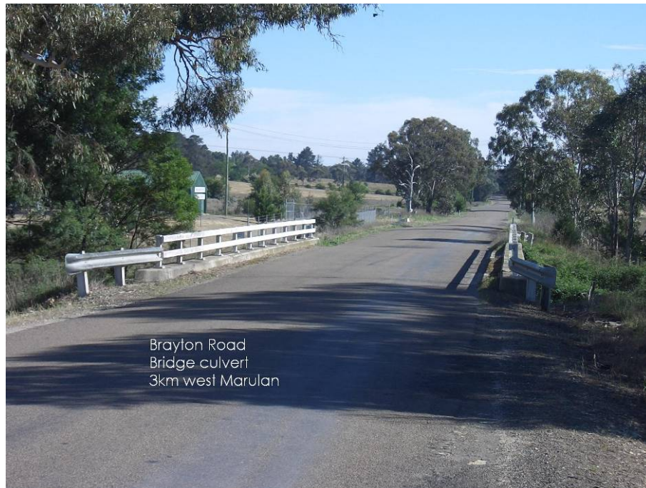
Figure 2-1 Brayton Road showing narrowing over bridge culvert
