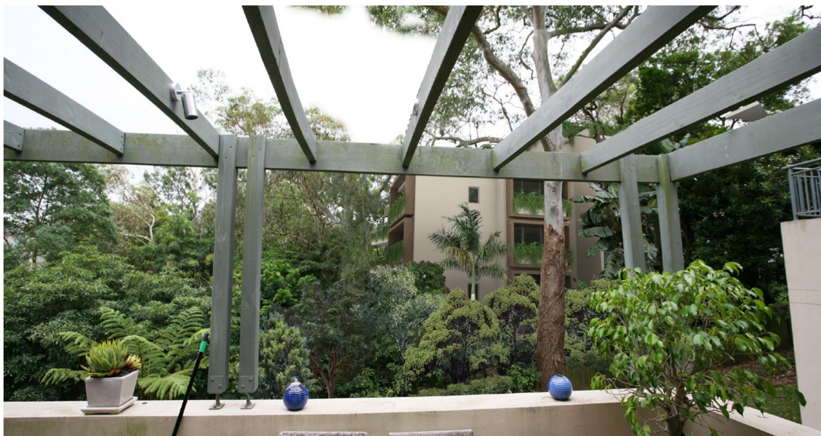
Alternative Envelope At Completion
