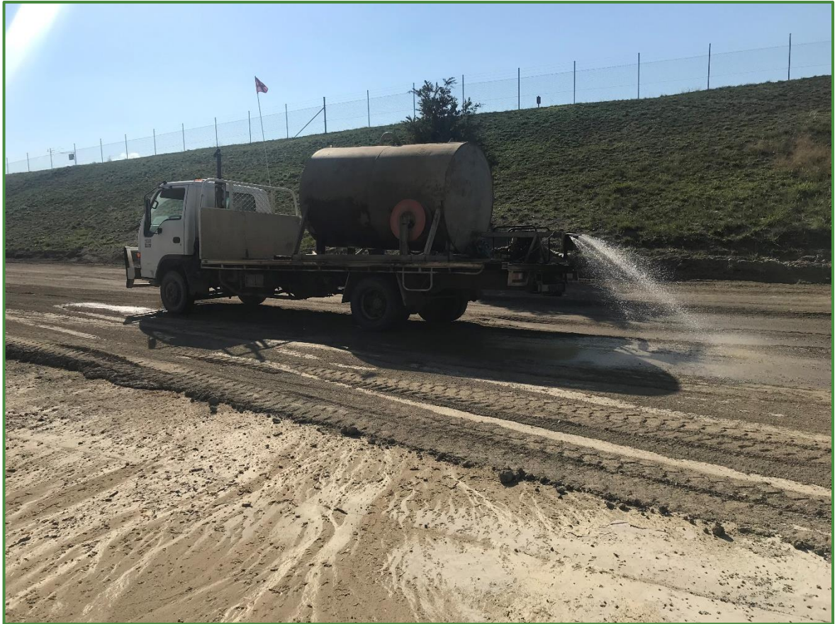
Figure 1-1: Watercart containing “Dustex” providing dust suppression to the site
