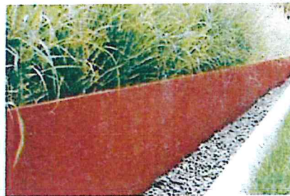
USBS - CD: 01 - Corten Steel retaining walls
