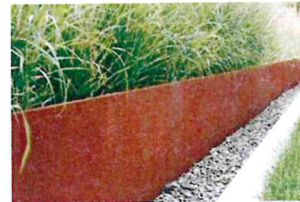
USBS - CD: 01 - Corten Steel retaining walls
