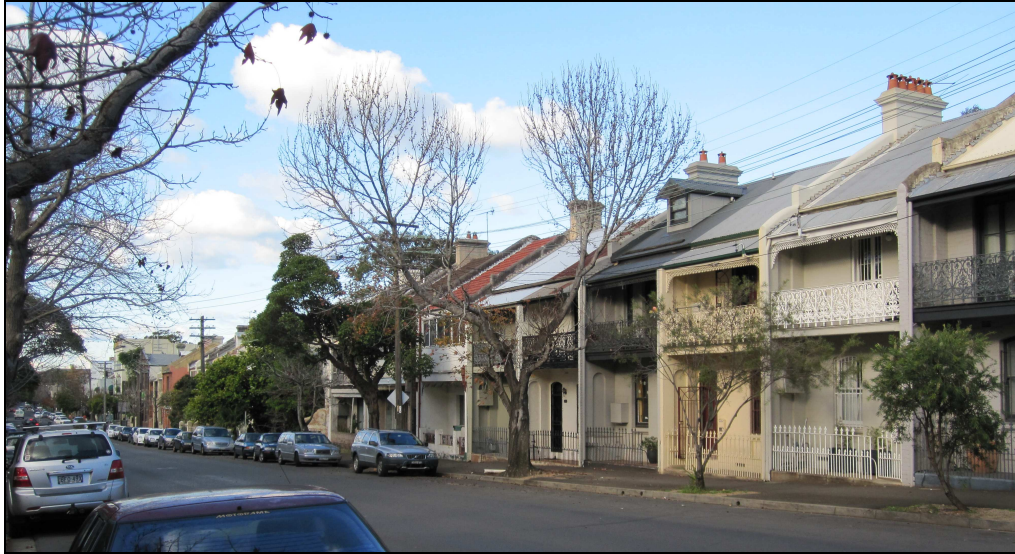
Figure 4: Existing Abercrombie Street residential terraces
