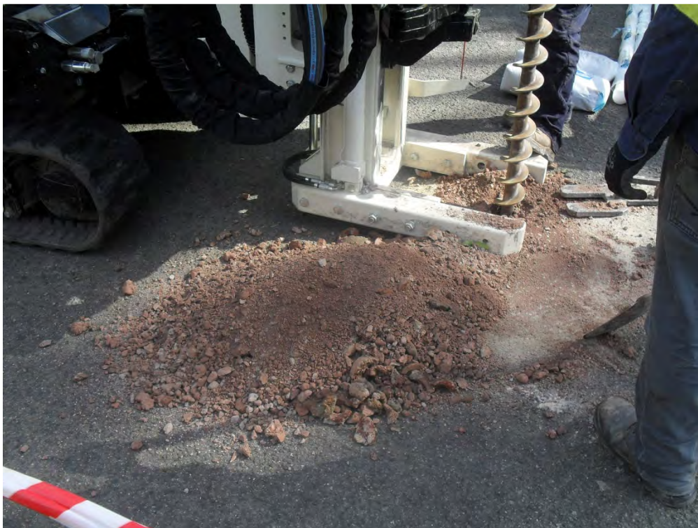
Photo 8 Soil Material found at MW02.
