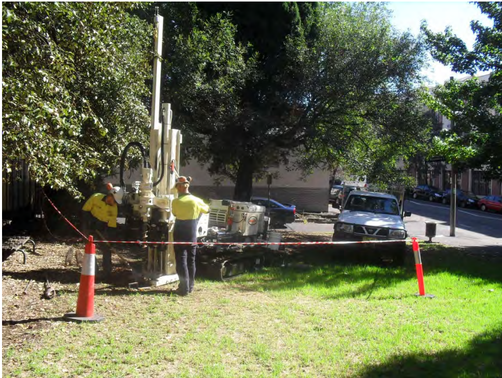
Photo 9 Rig set up for pushtube drilling for MW03.
