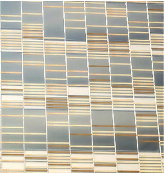
USBS - CL: 02 - Terracotta screen : Solar protection treatment to glazing system
