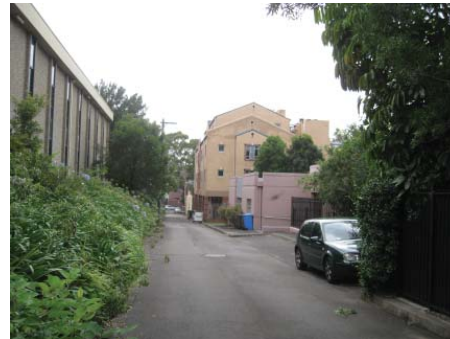
Boundary Lane - Mandelbaum House retained.
