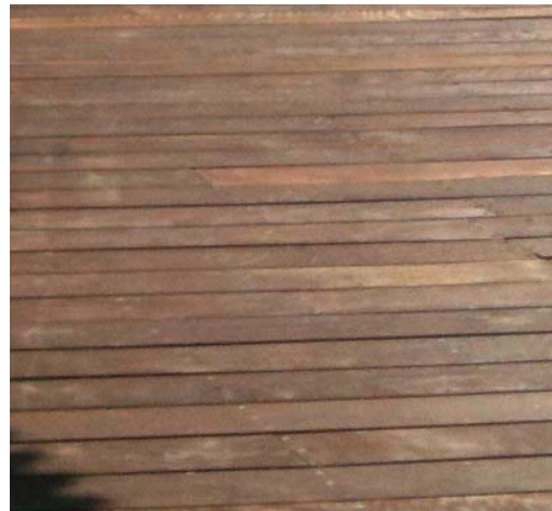
Timber decking - Spotted Gum
