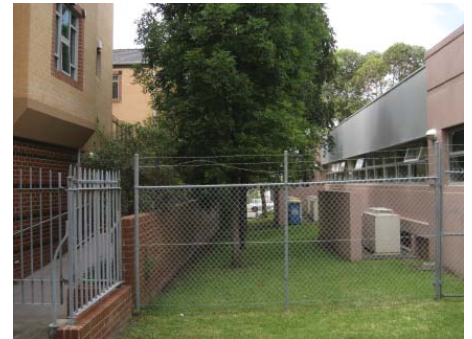
Basement access for new Business School.
