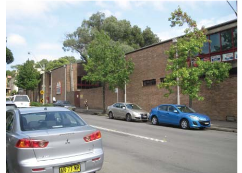
Shepherd House demolished.
