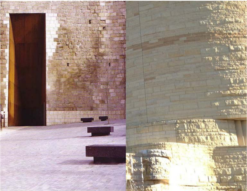
USBS - CD: 02 - Sandstone retaining walls and external walls
