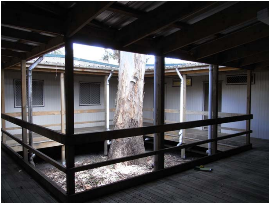
Photograph 1: Tree # 1 - Illustrating the location of the tree within the area of demountable buildings facing Codrington Street.
