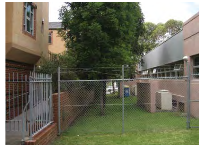
Basement access for new Business School.
