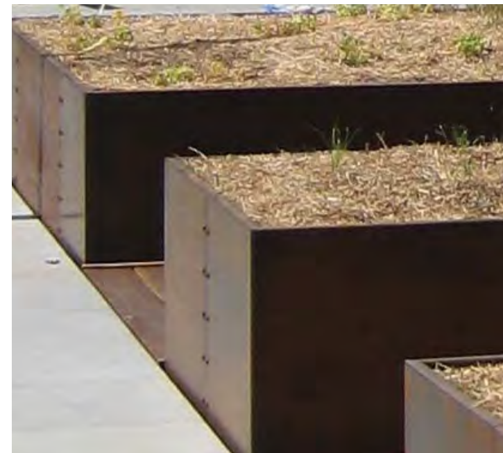
Corten planters - folded 3mm Corten sheets on galvanised steel frame
