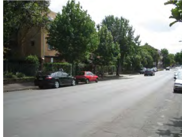
Mandelbaum House to the East retained.
