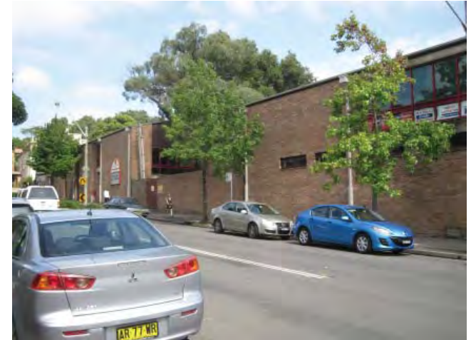
Shepherd House demolished.
