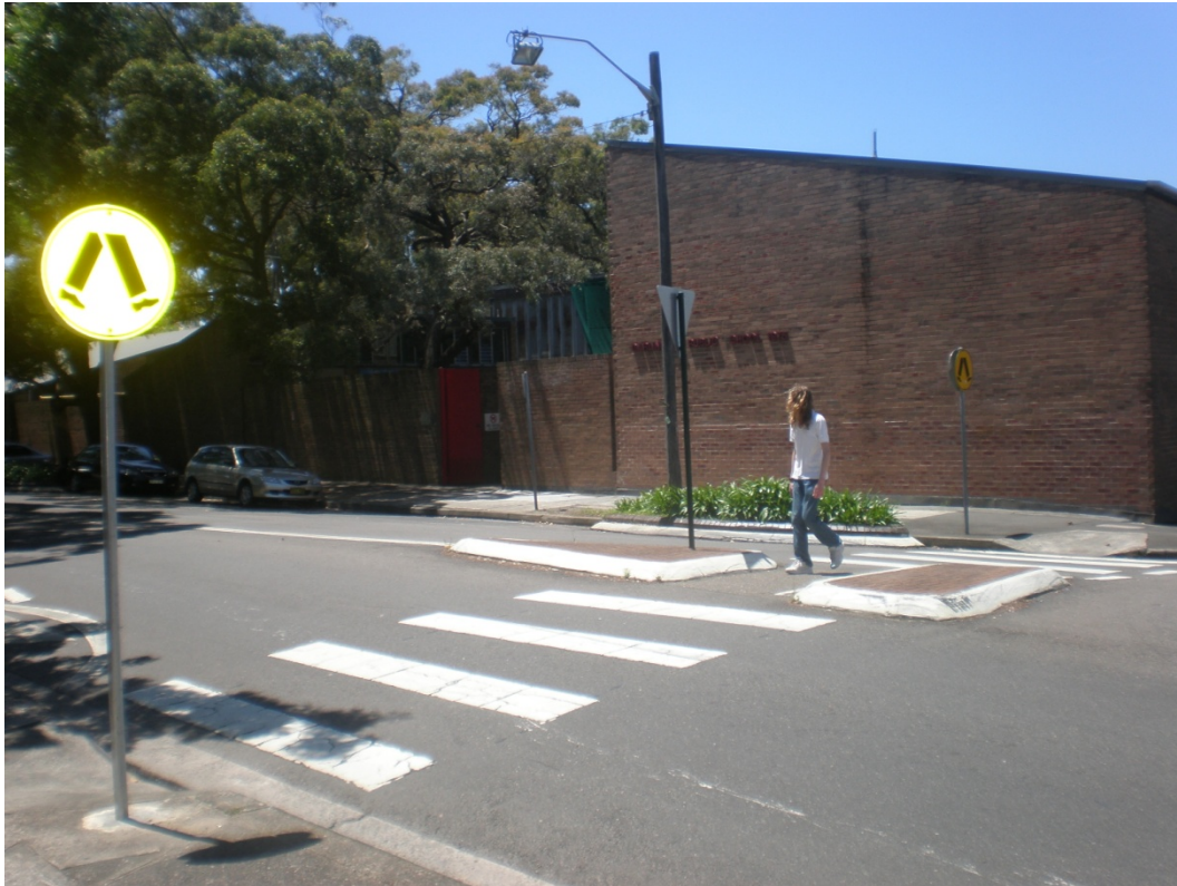
Photograph 5 Pedestrian crossing on Golden Grove Street
