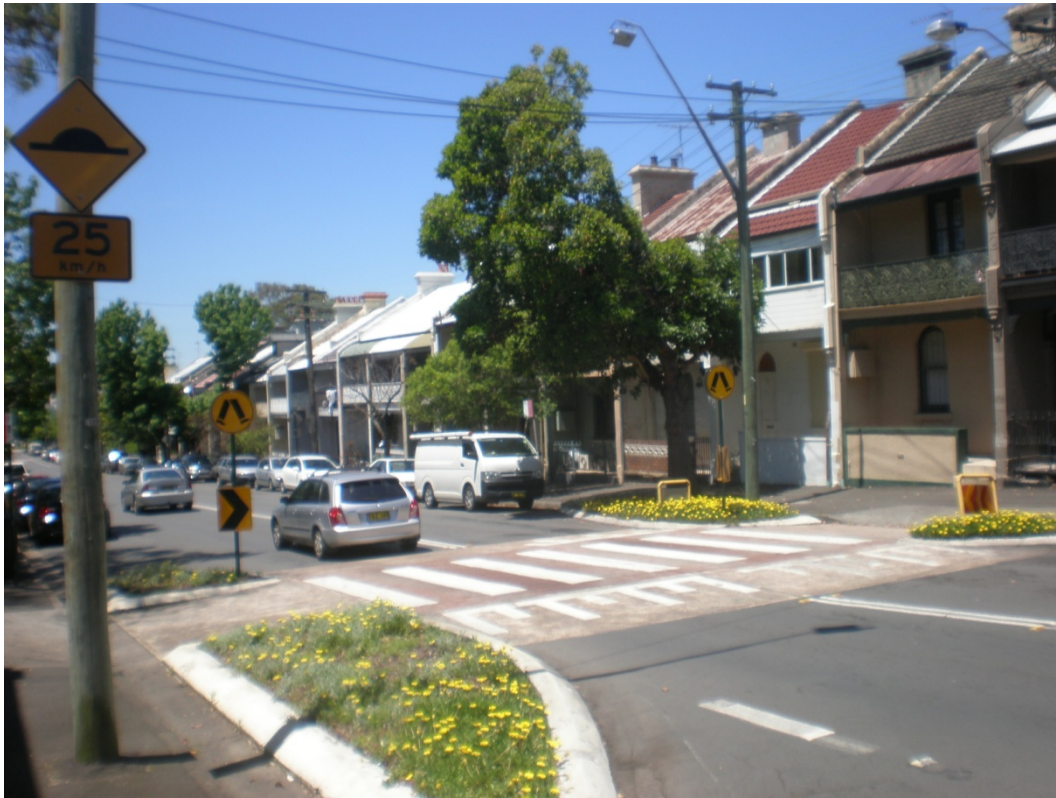
Photograph 2 Raised pedestrian crossing on Abercrombie Street
