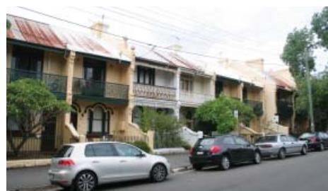
Figure 3.8: Darlington Road terraces
