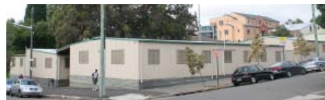
Figure 3.17: Geology Department demountables, at the corner of Codrington Street and Boundary Lane
