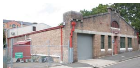
Figure 3.15: Joiner's Workshop (proposed for demolition), main Rose Street facade
