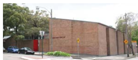
Figure 3.5: Darlington Public School looking from corner of Golden Grove & Abercrombie Street
