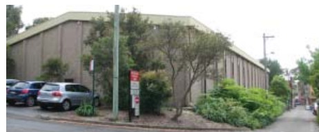
Figure 3.16: Clark Building and Boundary Lane, looking east
