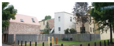
Figure 3.10: Rear of terraces looking from corner of Codrington Street and Darlington Lane
