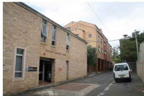
Figure 3.18: University Computing Centre and Boundary Lane, looking west
