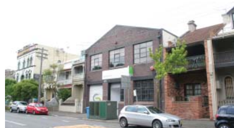
Figure 3.4: Row of terraces across Abercrombie Street, to the south of subject site, looking east
