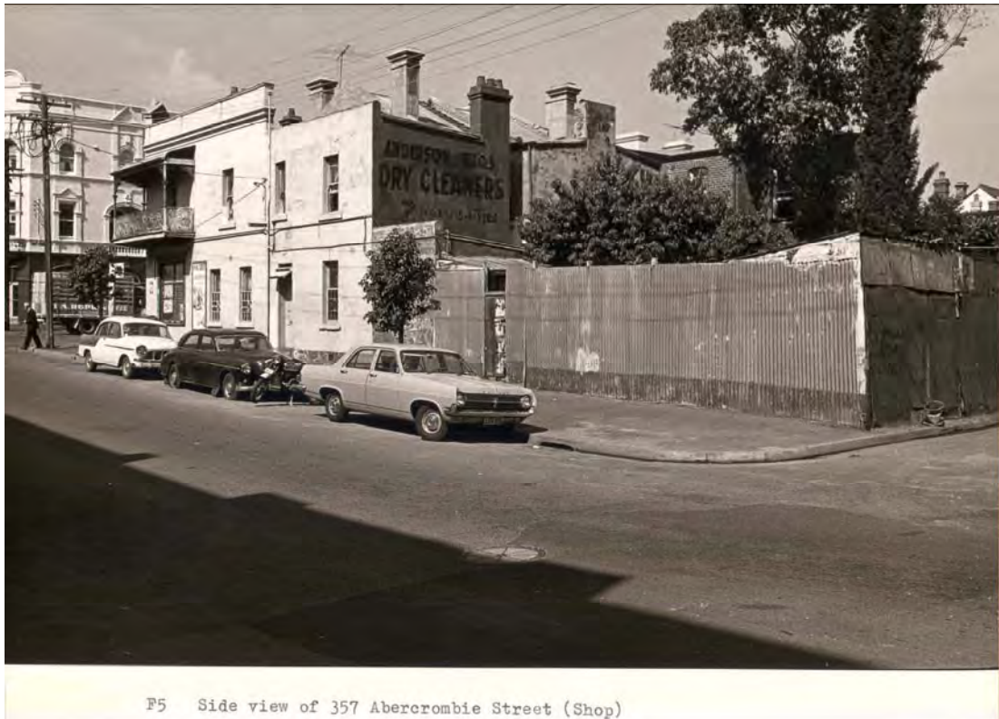
Figure 2-13: View of the corner of Codrington and Abercrombie Streets, taken from Codrington. This corner shop and the adjoining property are now a small park (Area 8), Fig. 1-5. SU Archive F5.
