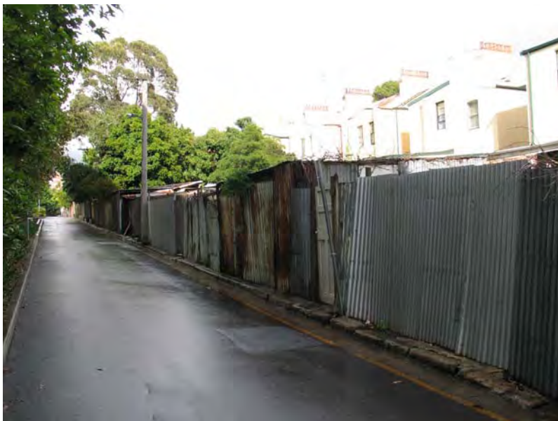
Figure 1-9: Area 5, Darling Lane, looking west, midway along the laneway, rear yards of Darlington Road Houses. This photo was taken mid-way along the laneway in Figure 1-8.
