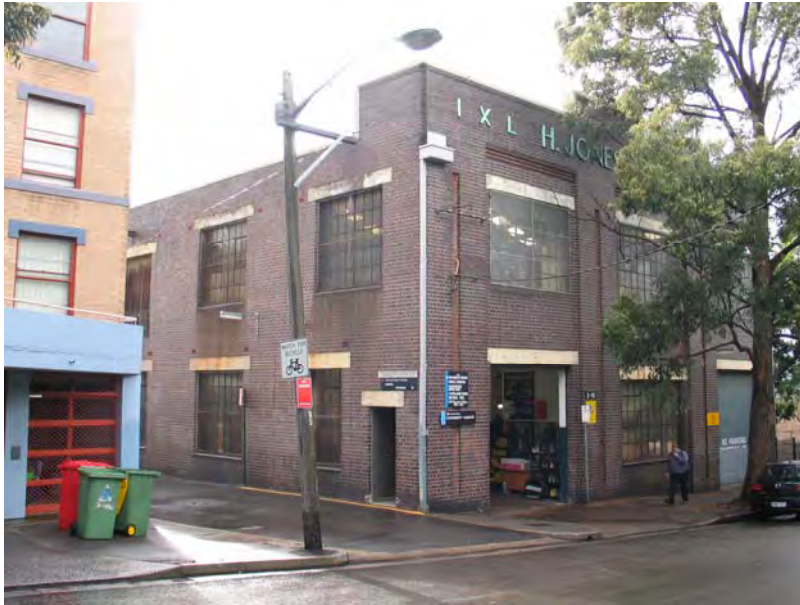
Figure 1-11: Area 5, western end of the study area with Darlington Lane and the University Garage, former IXL House (right) to the south.
