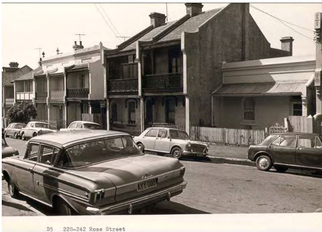
Figure 2-12: View of 228 to 242 (190 to 202 on the 1892 plan) Rose Street south, within Area 6. This photo shows cottages and terraces, some semi-detached, and a single-storey semi at 242. SU Archives D5.
