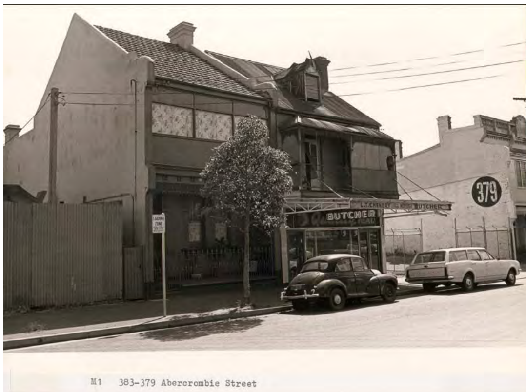
Figure 2-14: Photo of 383 to 379 Abercrombie Street (280 to 274 on the 1892 plan), within Area 8. The carpark is no. 379 on Fig. 2-8. This photo illustrates the more mixed residential and commercial nature of Abercrombie Street to either Darlington Road or Rose Street. SU Archives M1.
