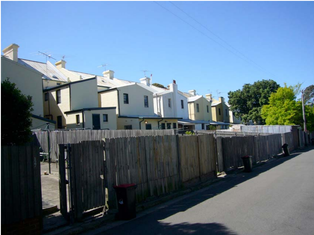
Figure 12 – Darlington Lane – rear of terraces
