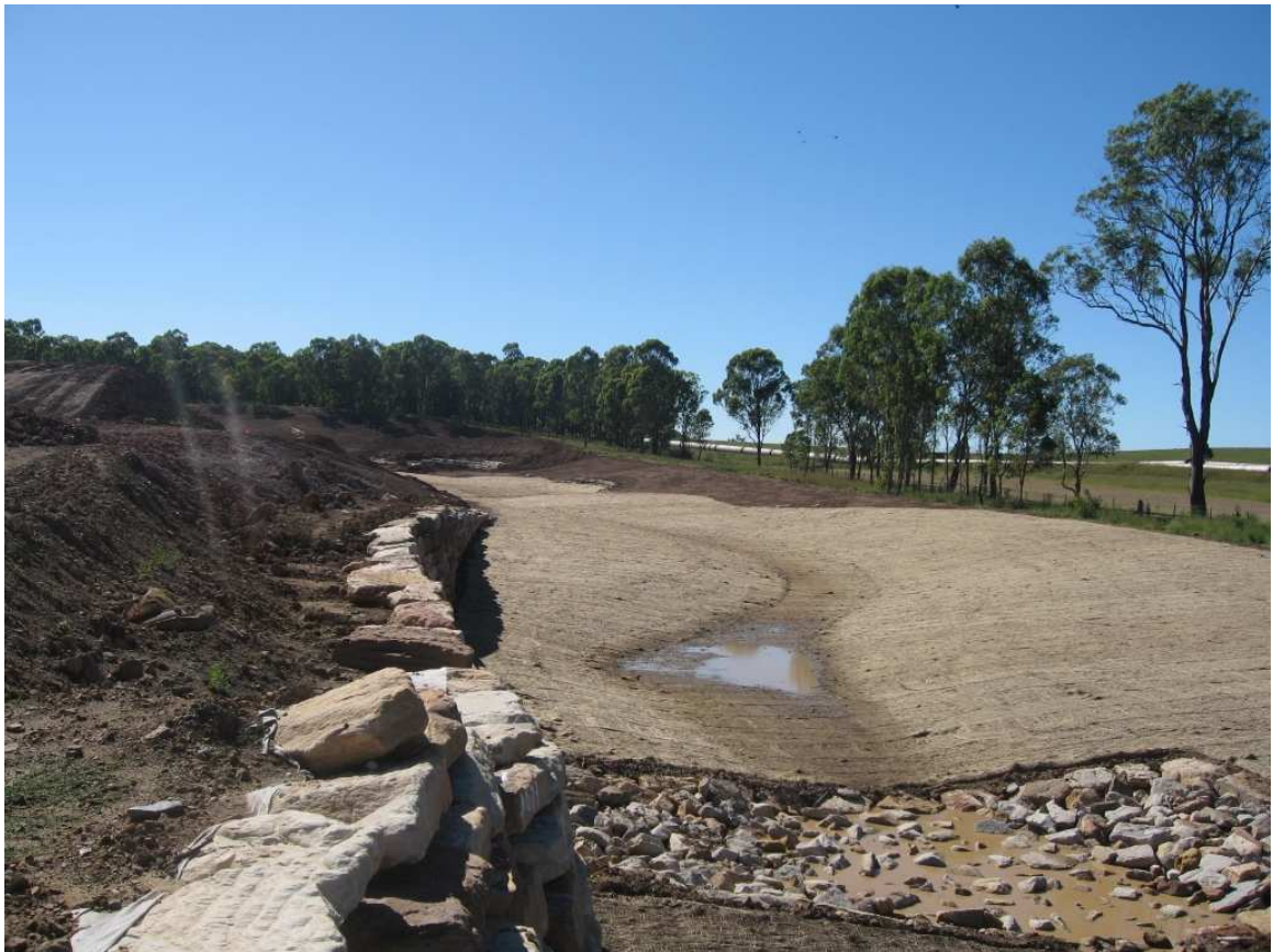
Photo 2 The CSR watercourse upstream from the proposed crossing. The eastern end of the subject site is visible to the right of the constructed watercourse, extending to the Sydney water pipeline.
