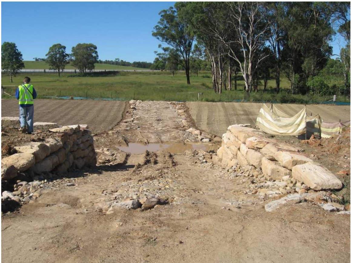
Photo 1 Site of proposed crossing over the constructed watercourse on the CSR lands. The western end of the subject site is located beyond the watercourse, with the Sydney water pipeline in the background.
