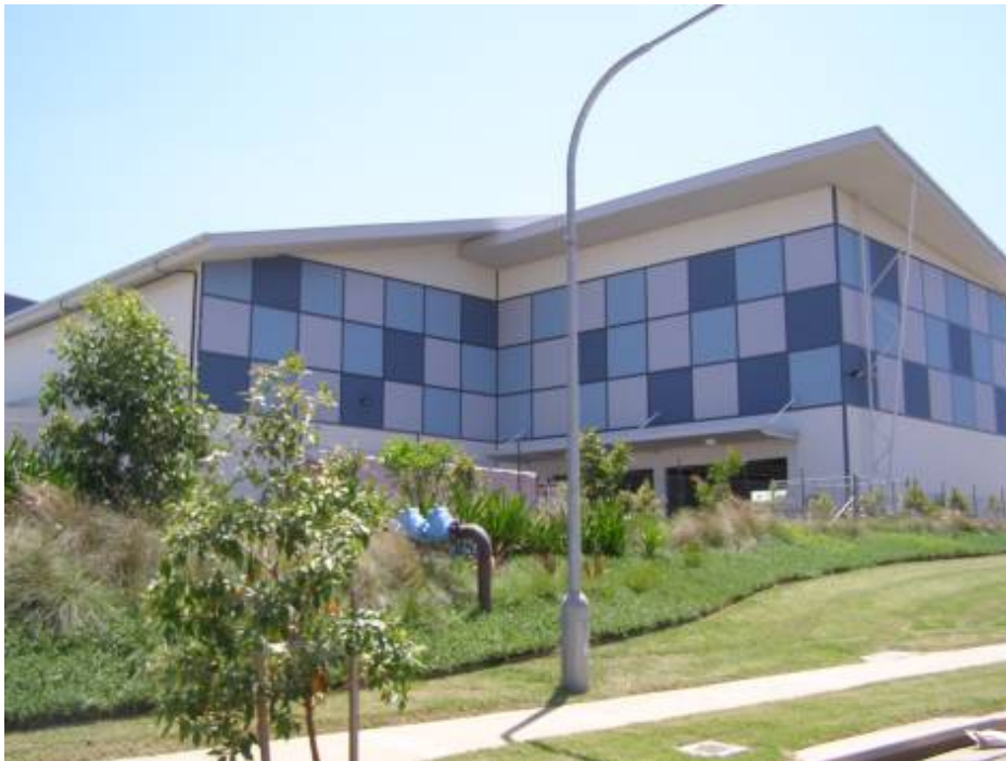
Figure 10 – BlueScope Steel (eastern facade fronting Templar Road)
