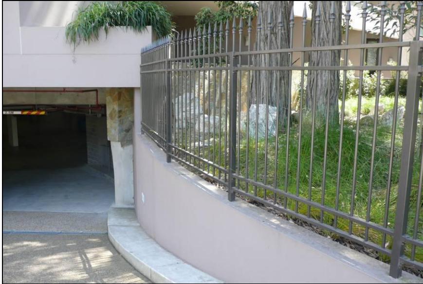
Photo E: Mature Turpentine within 3 metres of basement construction adjacent multi-storey development at 1 Newhaven Place St Ives.
