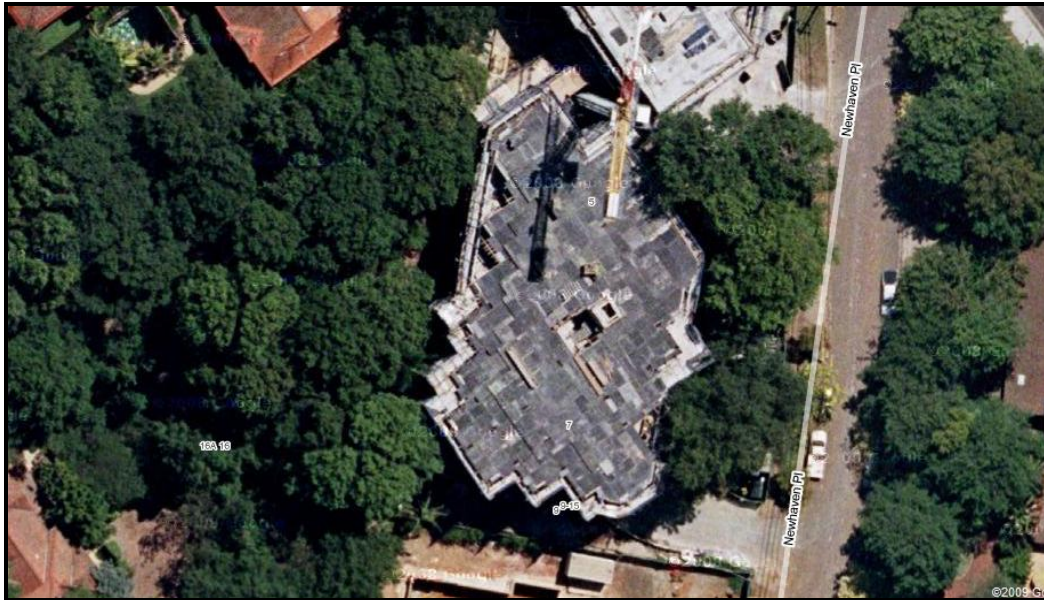
Photo G: Aerial photo of 1 Newhaven Place partially completed showing proximity of building to existing forest.
