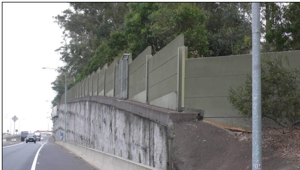
Photo B: Mature BGHF tree species surviving adjacent to construction on corner of M2 and Pennant Hills Road. The strip drains and weep holes behind the shotcrete wall have had no impact of existing trees.
