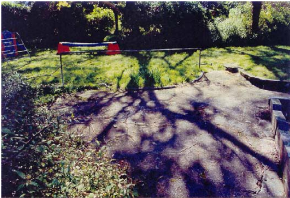
Figure 104: The western section of the original ‘potting garden’, now on the boundary of the property. The sandstone edging and crazy-paved paths are original elements of the garden layout (Mayne-Wilson & Associates, August 2000).
