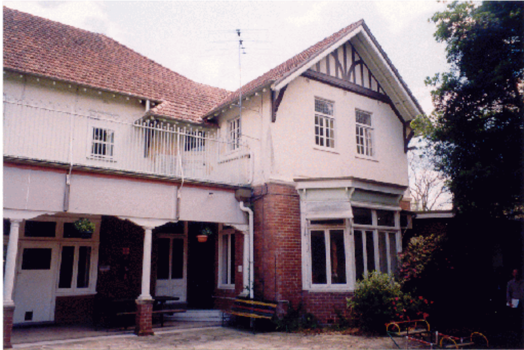
Figure 31: The eastern side of “Rippon Grange”. Modifications in this part of the house include the addition of lavatory facilities along the northern corner and replacement of early timber balustrades and shingle skirts associated with the first floor terrace with unsympathetic metal balustrading (Rod Howard Heritage Conservation Pty Ltd, October 2000).
