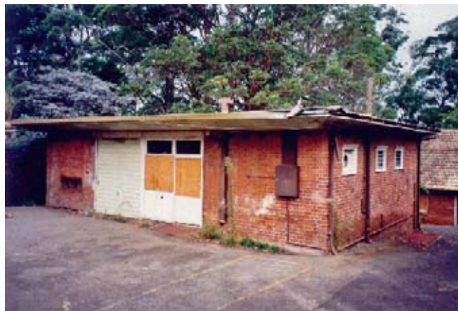
Figure 65: Although the Garage is amongst the earliest buildings on the site, it has been extensively altered over the years. The original gabled roof form has been replaced by this unsympathetic flat roof (Rod Howard Heritage Conservation Pty Ltd, October 2000).
