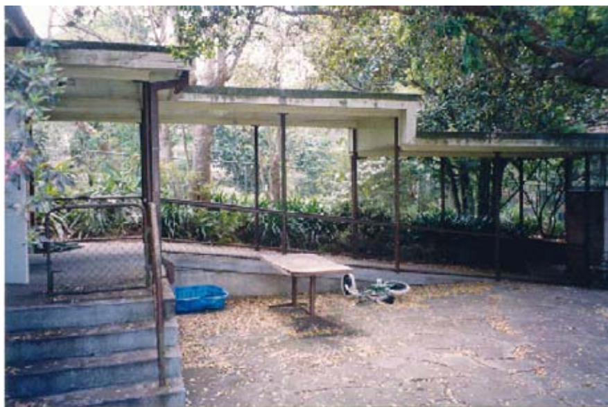
Figure 71: The covered way, constructed some six years later than the Playroom/Classroom, is rather more intrusive (Rod Howard Heritage Conservation Pty Ltd, October 2000).
