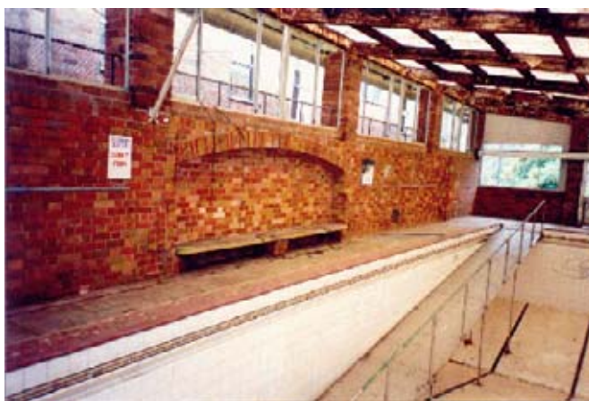
Figure 62: Early brick wall on the northern side of the Swimming Pool (Rod Howard Heritage Conservation Pty Ltd, October 2000).
