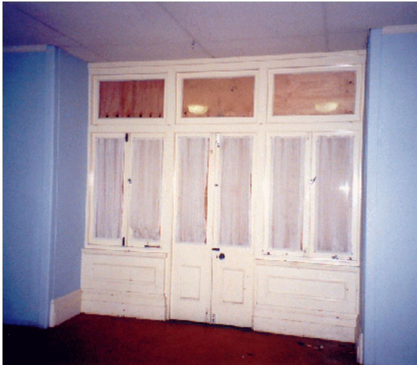
Figure 45: Early timber door and window joinery, eastern side of Room G14 (Rod Howard Heritage Conservation Pty Ltd, October 2000).
