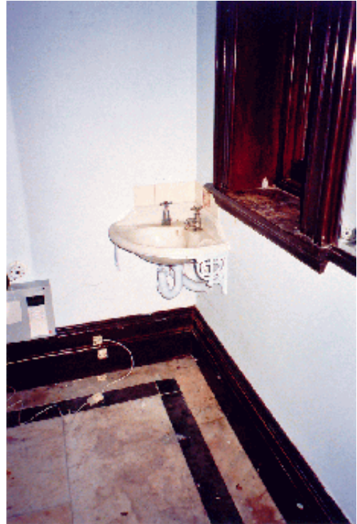
Figure 39: Flooring and lavatory basin in Room G2 (Rod Howard Heritage Conservation Pty Ltd, October 2000).
