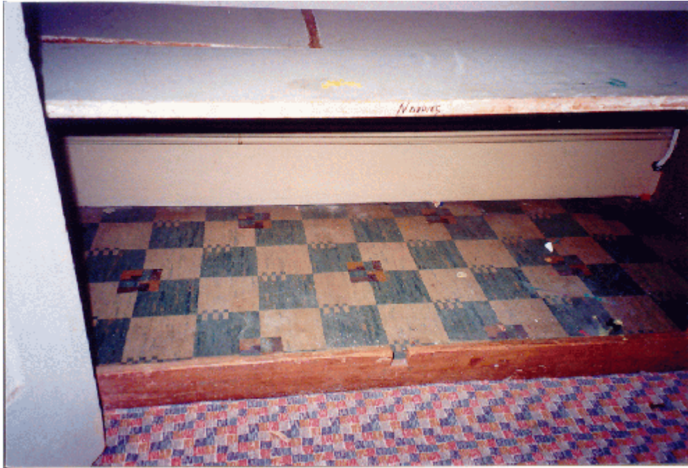
Figure 52: Circa 1935 linoleum on the floor of the cupboard on the southern side of Room F5 (Rod Howard & Associates Pty Ltd, 2005).
