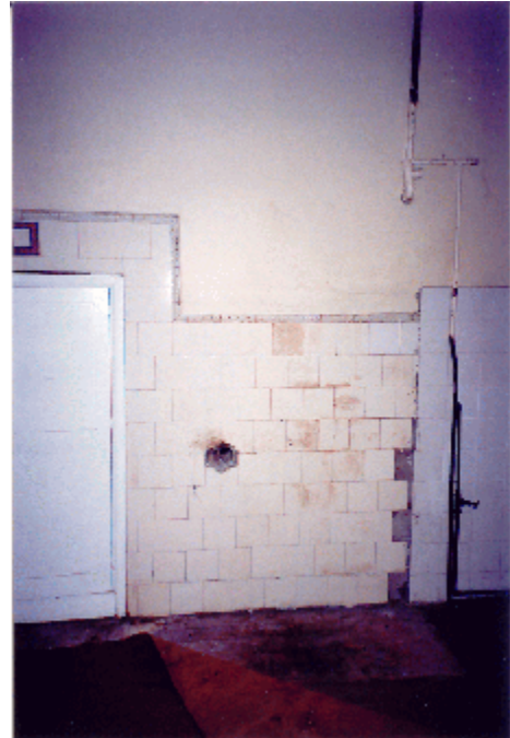
Figure 48: Tiling in Room G28, southern wall (Rod Howard Heritage Conservation Pty Ltd, October 2000).
