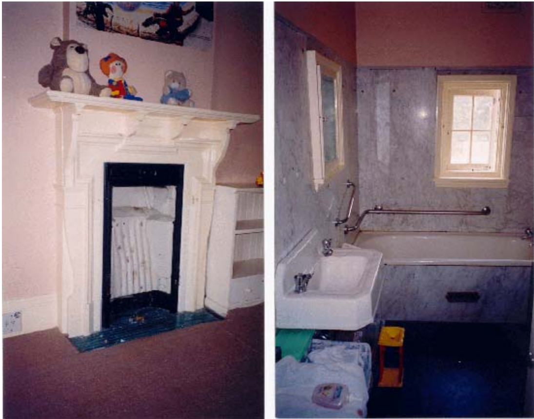
Figure 50: Important early fabric on the first floor of “Rippon Grange” includes this fire box and timber chimney piece in Room F3, at left, and the marble lining and metal bath vent in Room F4, at right (Rod Howard Heritage Conservation Pty Ltd, October 2000).
