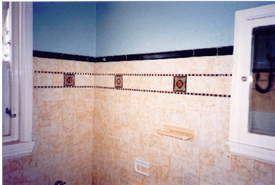
Figure 56: Circa 1935 wall tiling, Room F12 (Rod Howard Heritage Conservation Pty Ltd, October 2000).
