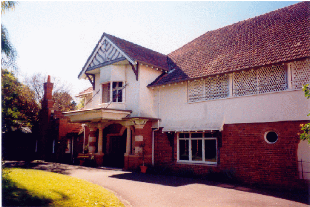
Figure 29: The western side of “Rippon Grange”. Although the exterior of the house has retained much of its early form and fabric, unsympathetic modifications include obscuring of verandahs and the replacement of timber shingle wall linings with a fire resistant plaster finish (Rod Howard Heritage Conservation Pty Ltd, October 2000).
