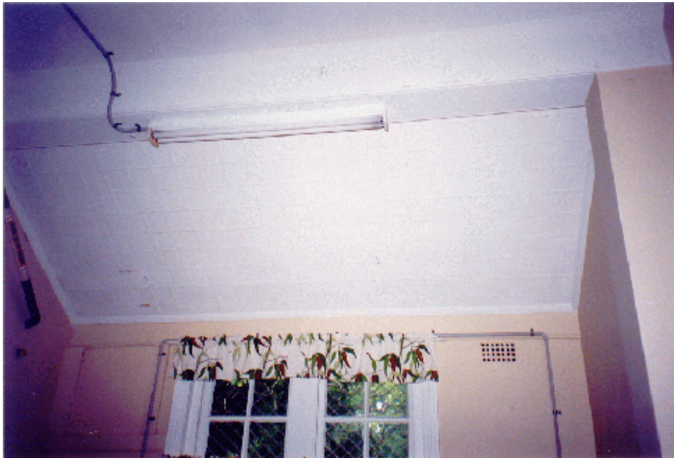
Figure 49: Pressed metal ceiling linings, western side of Room G28 (Rod Howard Heritage Conservation Pty Ltd, October 2000).
