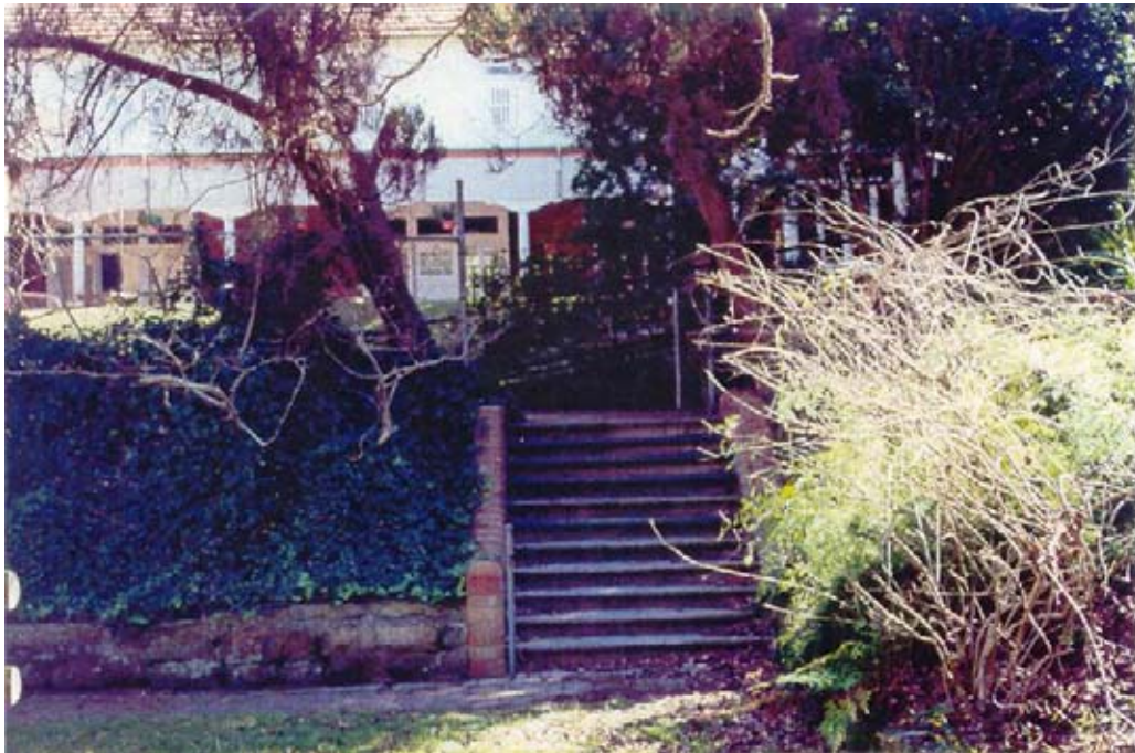
Figure 119: The main stairs leading between the original tennis court platform and the eastern forecourt to the mansion (Mayne-Wilson & Associates, August 2000).
