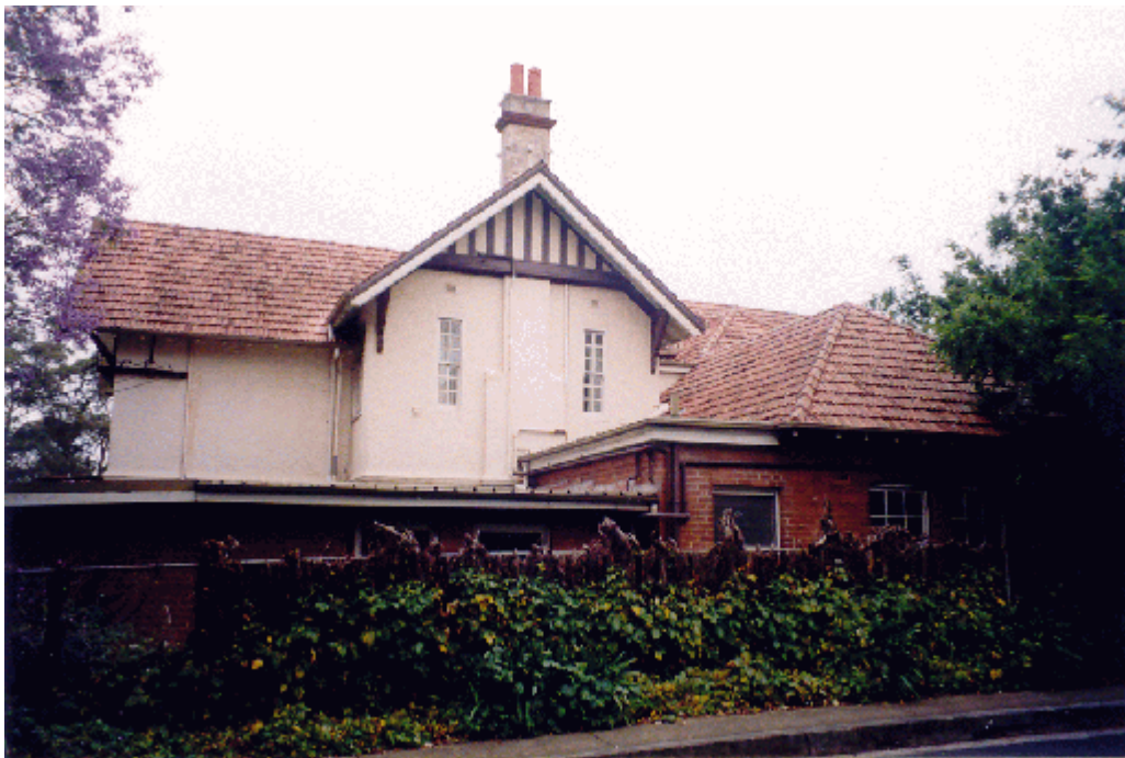
Figure 32: The northern side of “Rippon Grange”, with Howard Joseland’s addition of 1905 close to the street. Flat roofed additions dating from the 1950’s and 1960’s are also visible (Rod Howard Heritage Conservation Pty Ltd, October 2000).
