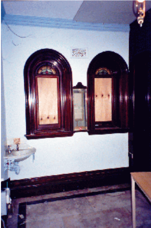
Figure 38: Western end of Room G2 (Rod Howard Heritage Conservation Pty Ltd, October 2000).
