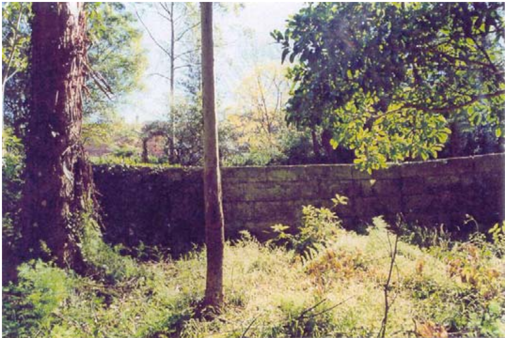
Figure 128: The eastern wall of the croquet lawn, closer to the northern end of the field. Glimpses of the mansion's roof are visible in the background of the photograph (Mayne-Wilson & Associates, August 2000).
