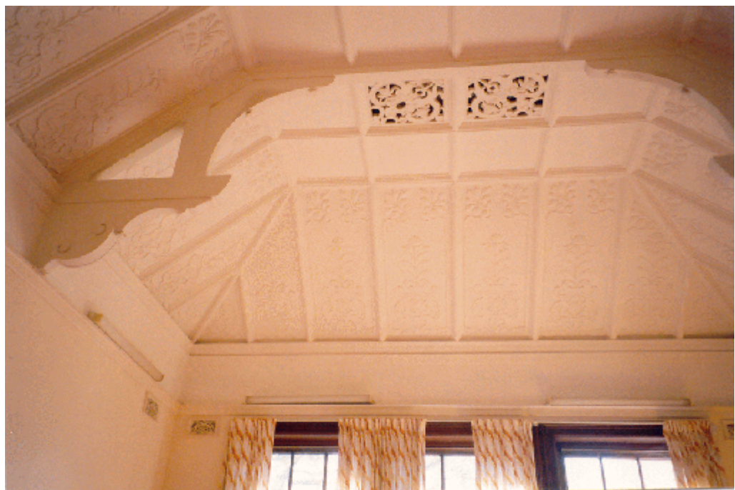
Figure 42: Intact original and early fabric in “Rippon Grange” includes the tiled paving of the eastern verandah floor, shown above, and the ceiling of Room G4, the 1905 billiard room designed by Howard Joseland, shown below (Rod Howard Heritage Conservation Pty Ltd, October 2000).
