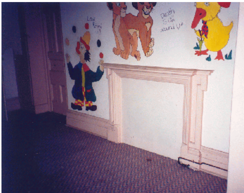
Figure 46: Fireplace joinery, northern wall of Room G15 (Rod Howard Heritage Conservation Pty Ltd, October 2000).
