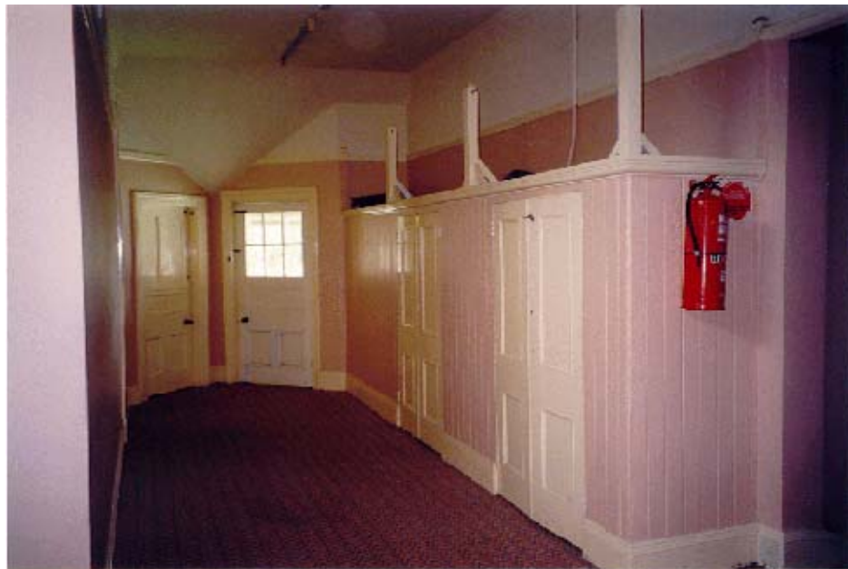
Figure 51: Early timber cupboards in corridor F5 (Rod Howard Heritage Conservation Pty Ltd, October 2000).
