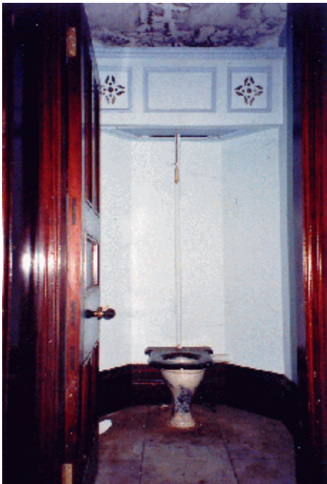
Figure 40: Water closet and cistern, Room G3 (Rod Howard Heritage Conservation Pty Ltd, October 2000).
