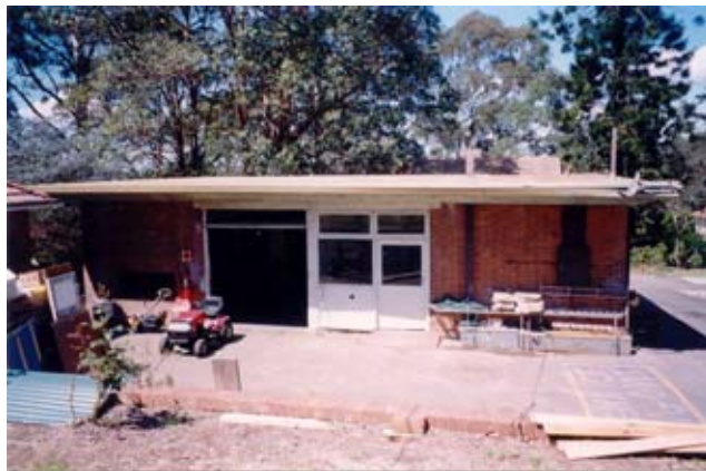
Figure 65: Although the Garage is amongst the earliest buildings on the site, it has been extensively altered over the years. The original gabled roof form has been replaced by this unsympathetic flat roof (Rod Howard Heritage Conservation Pty Ltd, October 2000).
