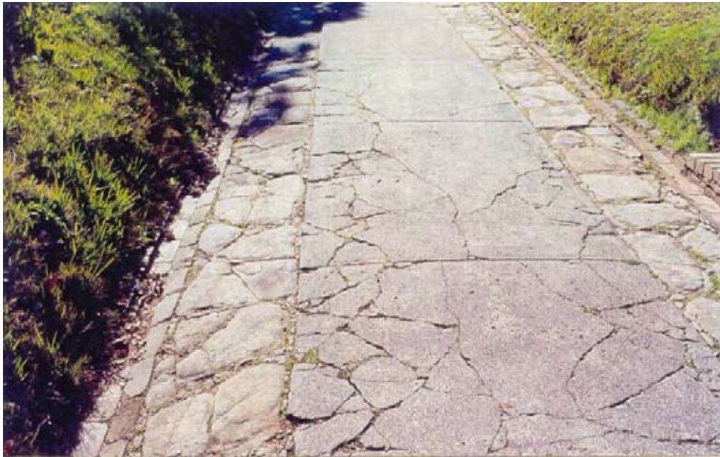
Figure 100: The concrete and sandstone driveway leading from the southern side of the mansion past the conservatory and ‘potting shed’. This may have originally been a service driveway to the kitchen area of the house. Note the brick spoon drains on either side of the driveway (Mayne-Wilson & Associates, August 2000).
