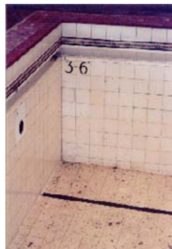
Figure 63: Tiling within the Swimming Pool (Rod Howard Heritage Conservation Pty Ltd, October 2000).
