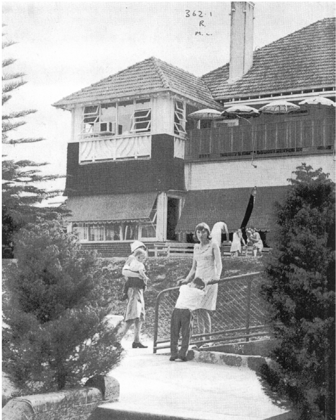
Figure 25: The south eastern corner of “Rippon Grange” prior to the addition of the 1970 ward block. The photograph was taken in the middle of the 1960's ( Eighty-Sixth Annual Report of the Royal Alexandra Hospital for Children, 1965-66, rear cover ).
