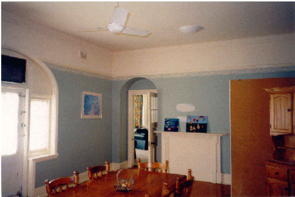
Figure 53: Room F10 has been modified to become living spaces, and finishes from the 1981 refurbishment are still in place (Rod Howard Heritage Conservation Pty Ltd, October 2000).
