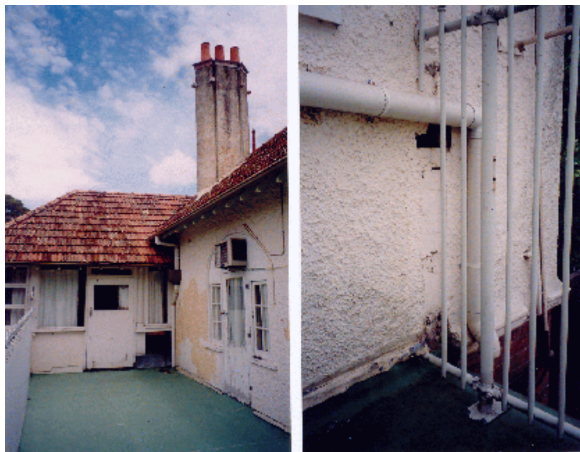
Figure 34: The open first floor terrace on the eastern side of “Rippon Grange” has been extensively modified. This includes enclosure of the loggia at the southern side of the terrace, modification of openings in the eastern wall of “Rippon Grange” and removal of original balustrades and handrails (left). An unsympathetic metal balustrade has been installed, along with insensitively placed rainwater goods, but evidence of the profiles of original balustrade and handrail joinery is still visible on wall surfaces (right) (Rod Howard Heritage Conservation Pty Ltd, October 2000).
