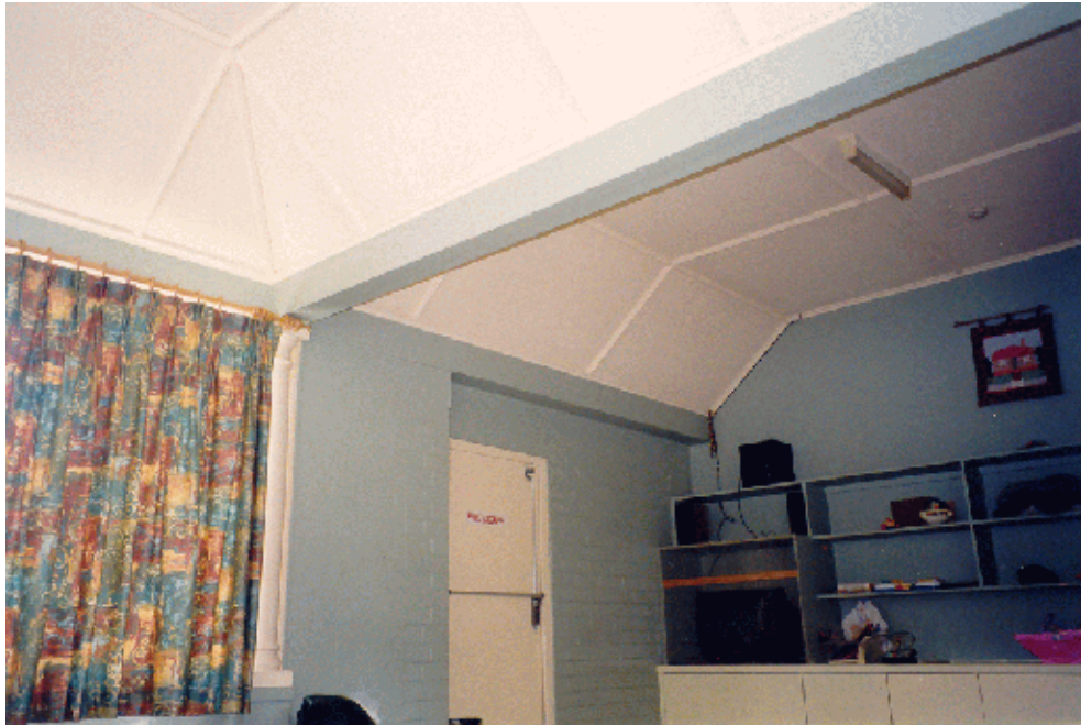
Figure 54: Room F11 was modified by the construction of the fire stair at the end of the 1950's (Rod Howard Heritage Conservation Pty Ltd, October 2000).
