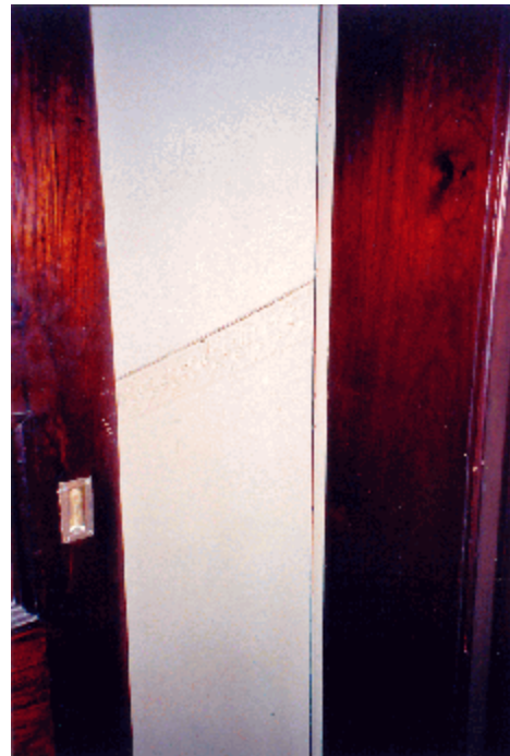
Figure 41: Early wall linings in the curved stair space off the south-western corner of Room G13 (Rod Howard Heritage Conservation Pty Ltd, October 2000).
