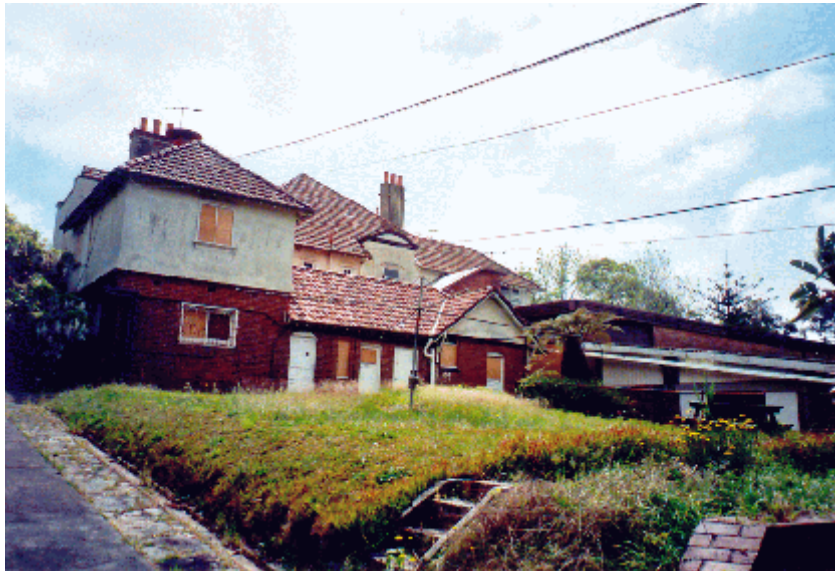
Figure 33: “Rippon Grange” viewed from the south, near the Garage (Rod Howard Heritage Conservation Pty Ltd, October 2000).
