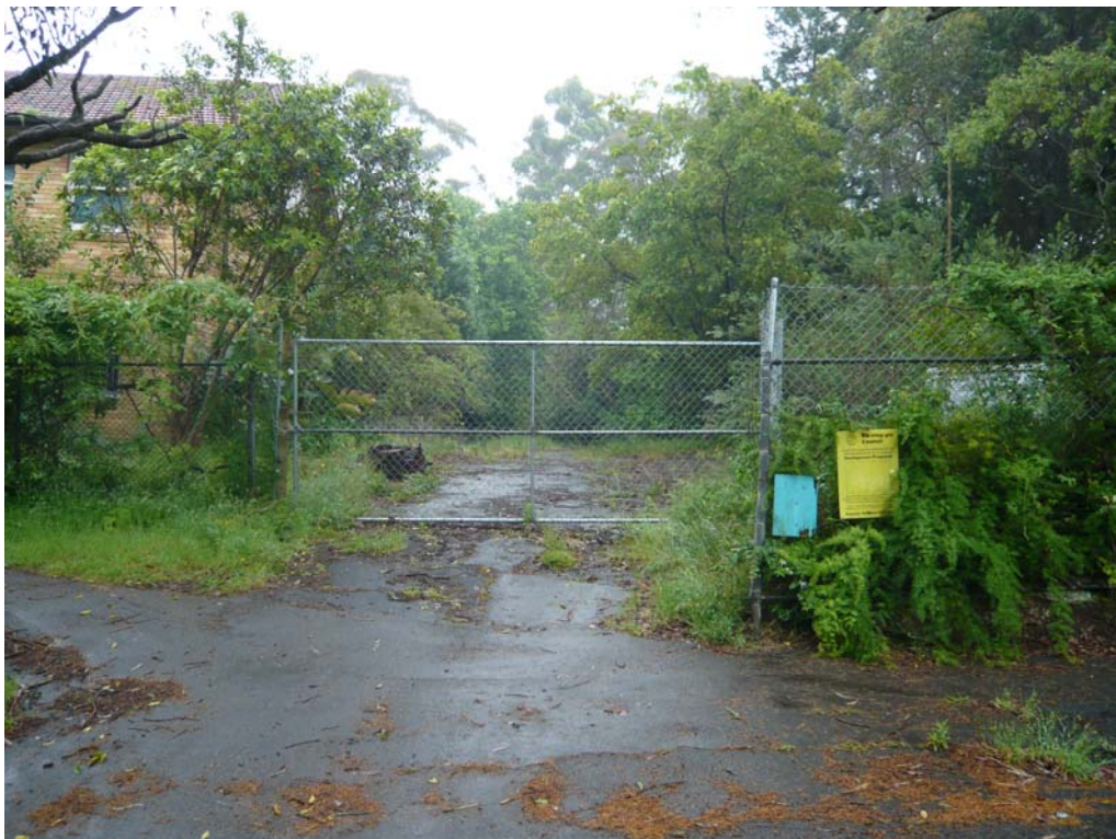
View of existing access onto Young Street.
