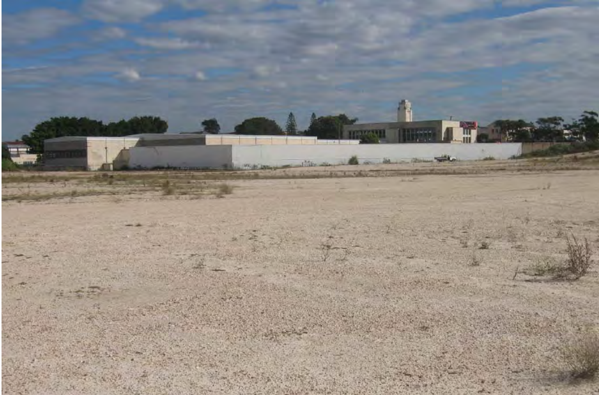
Figure 3.1 View to the west showing the large area of sandstone rubble fill located across the eastern half of the subject site. Note the c1959 constructed Penfolds Warehouse complex with its distinctive clock tower. The sandstone fill is likely to cap the fill of the quarry, associated with the former brickworks, which was located in this area of the site. (Source: GML 2008)
