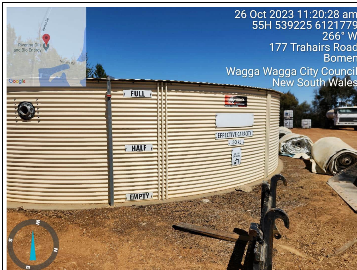
Photo 66: Firefighting water storage tank 1 - full
