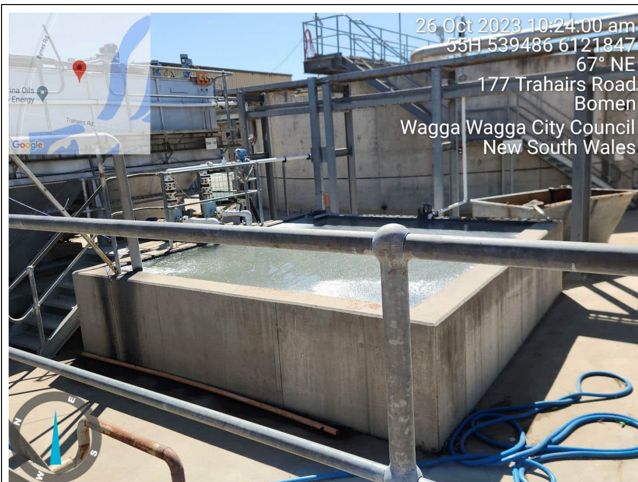
Photo 39: Wastewater treatment plant
