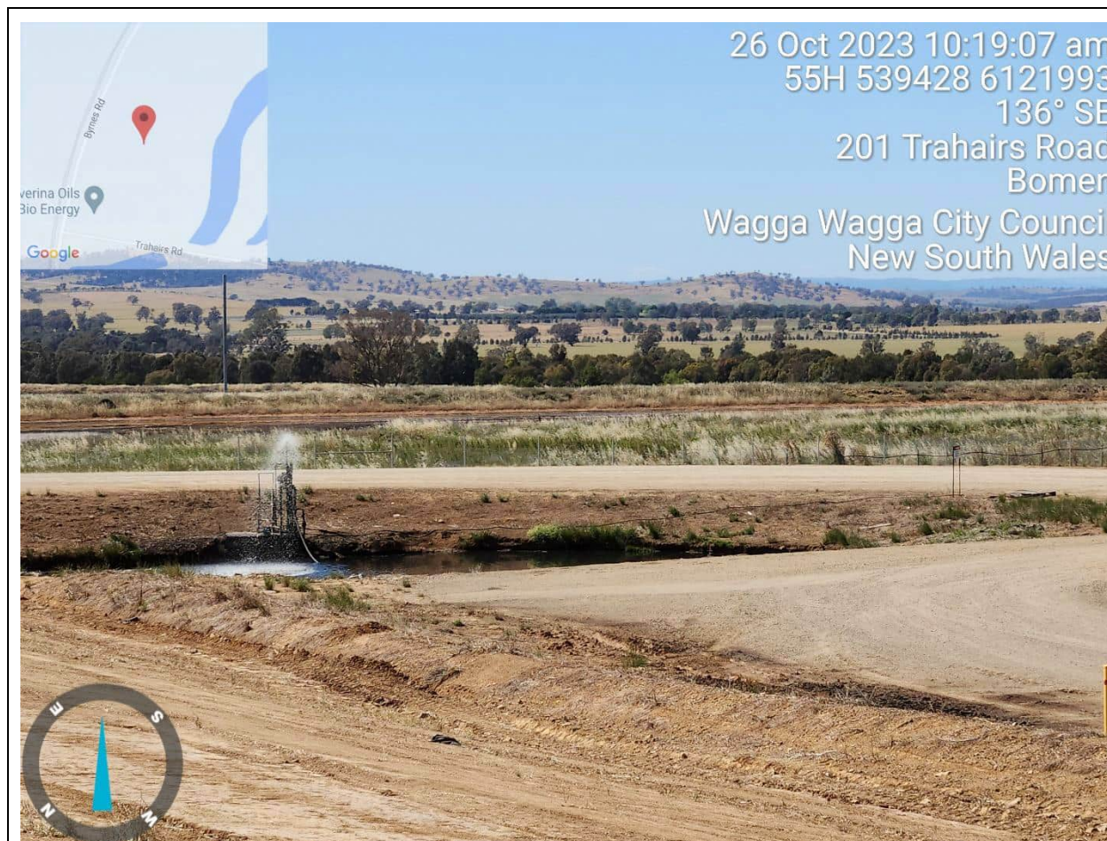
Photo 35: Stormwater control dam from bulk grain store
