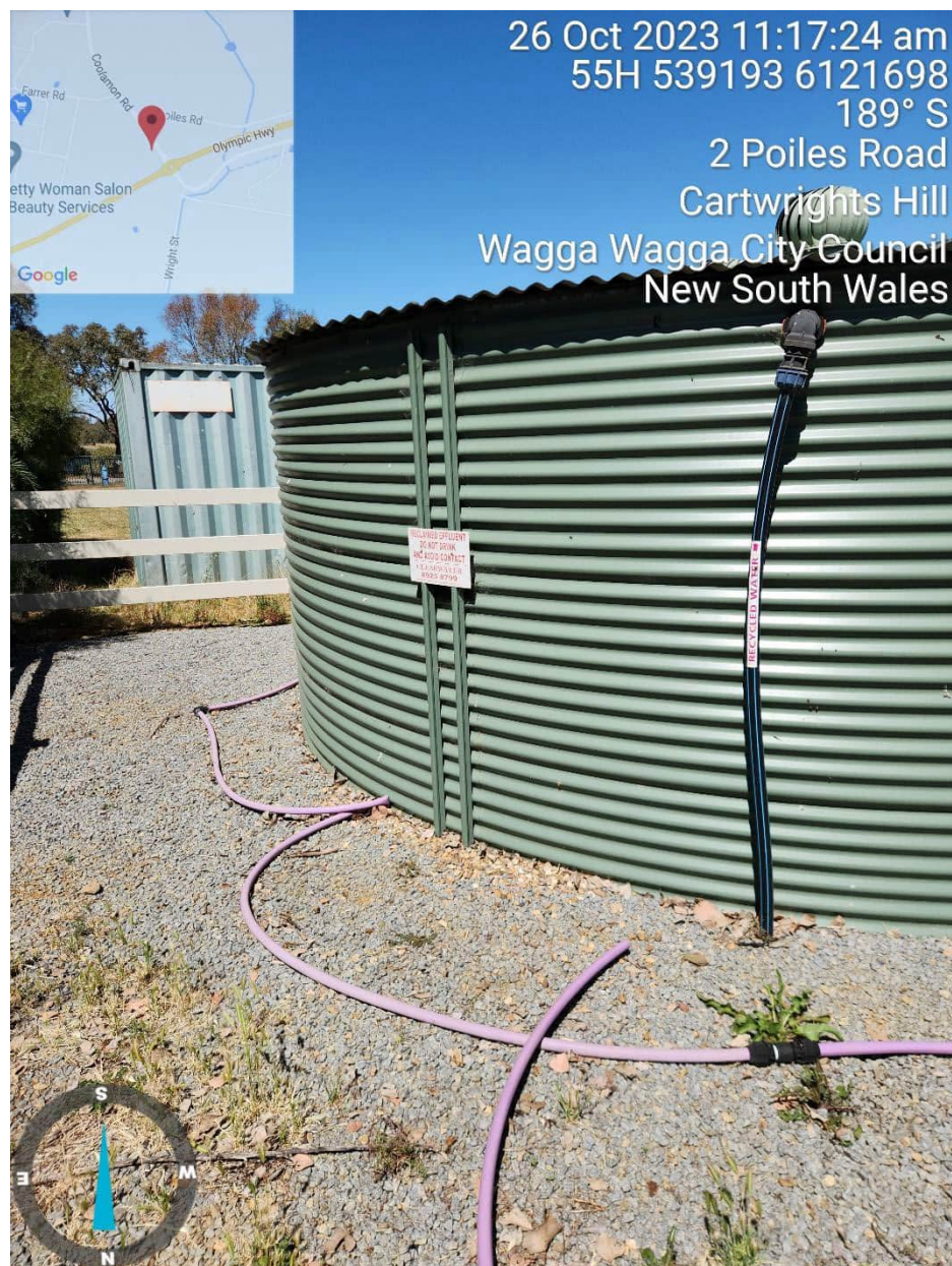
Photo 60: Treated effluent storage tank
