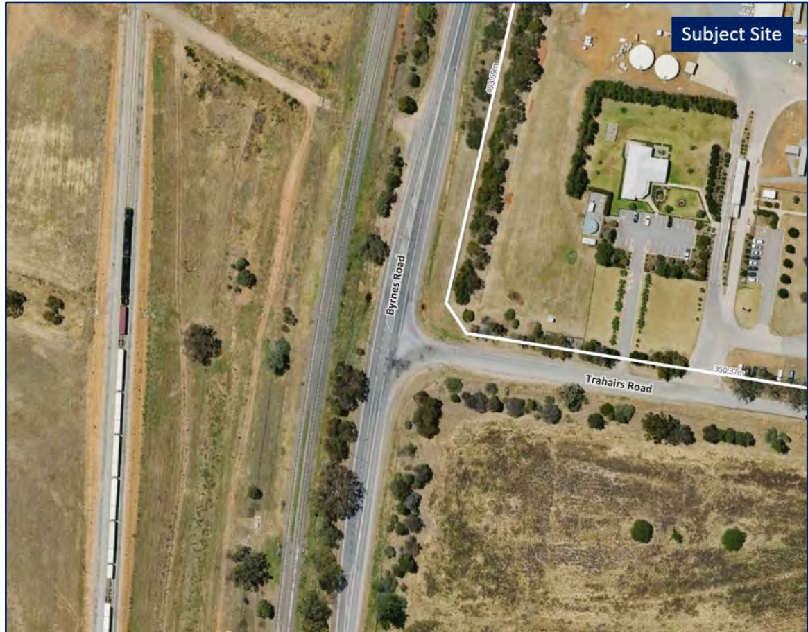
Figure 2.7: Brynes Road / Trahairs Road Intersection
