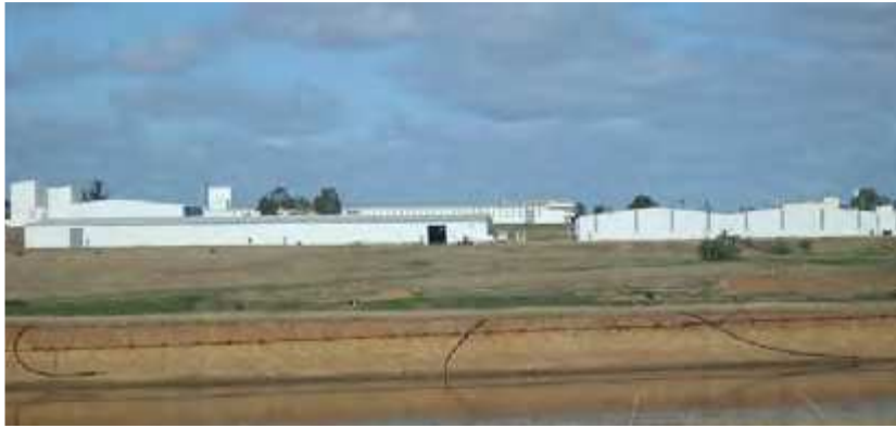
Figure 17: Existing Wool Combing Facility
