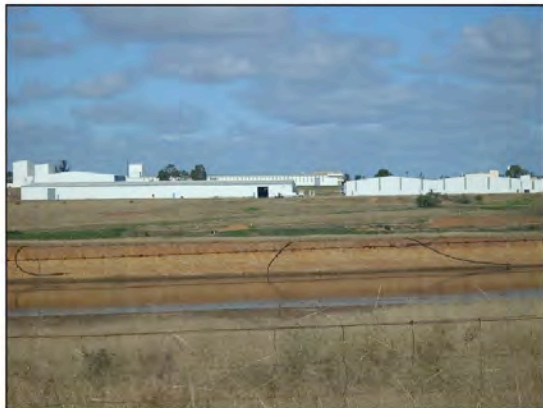
Image 3: Wool processing factory. The study site is adjacent to the already visually prominent industrial buildings.
